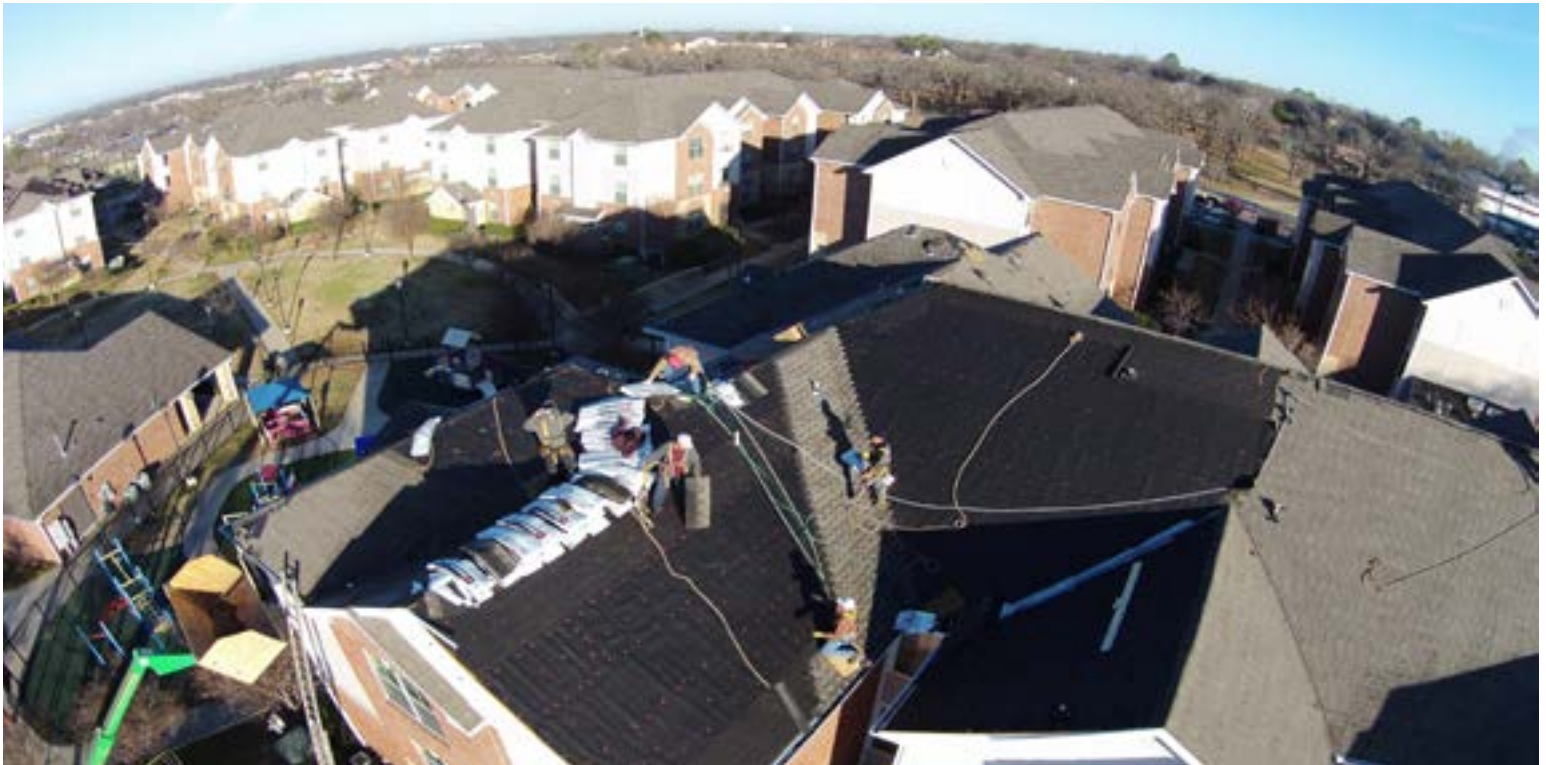
(Texas Woman's University Roofing Project)
