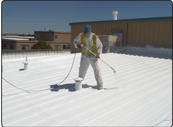
Spraying on Apoc 252 SunWhite (2 top coats used, sprayed perpendicular to each other)
