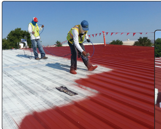
Spraying on Apoc 291 Rust Inhibitive Primer
