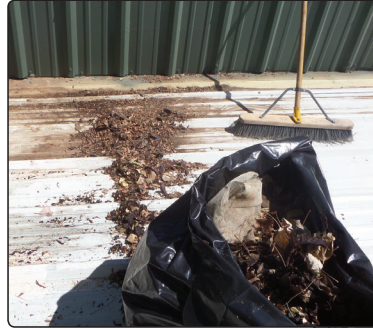
Preparing roof by clearing debris and pressure washing
