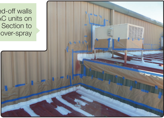
Spraying on Apoc 252 SunGrey Premium Elastomeric Roof Coating (2 base coats used, sprayed perpendicular to each other)
