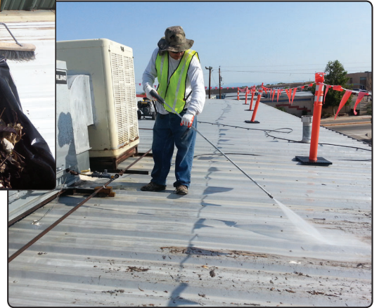
Preparing roof by clearing debris and pressure washing
