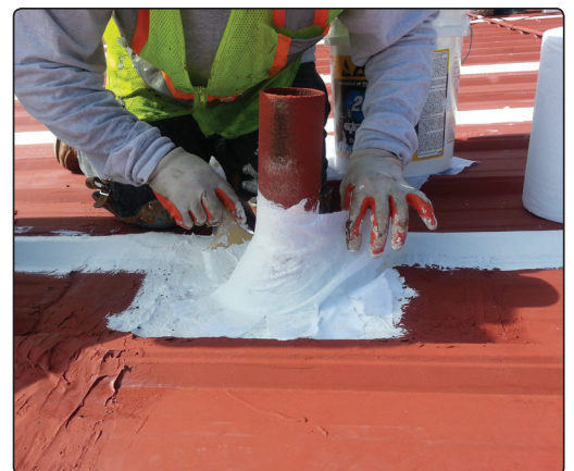
All perimeters, curbs and penetrations are sealed with Apoc 264 & reinforcing fabric
