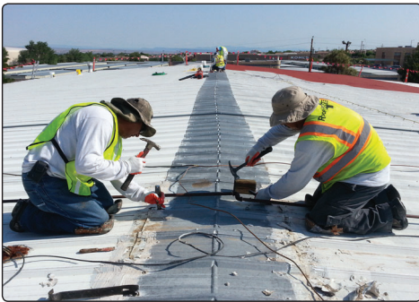
Removing old material used on previous repairs
