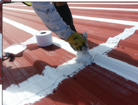
All perimeters, curbs and penetrations are sealed with Apoc 264 & reinforcing fabric
