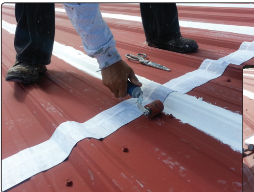
Sealing horizontal seams with Apoc Fleece-Top Incredible Repair Tape and Sealant, followed by Apoc 264
