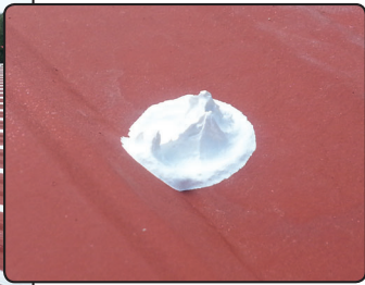
Sealing fasteners with Apoc 264
