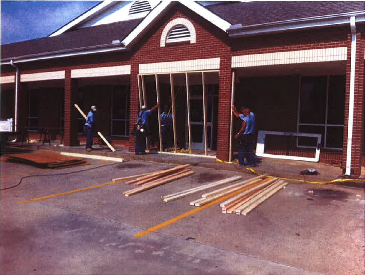
Vehicle Impact – Temporary board up prior to permanent repair – Chenal Post Office 2011
