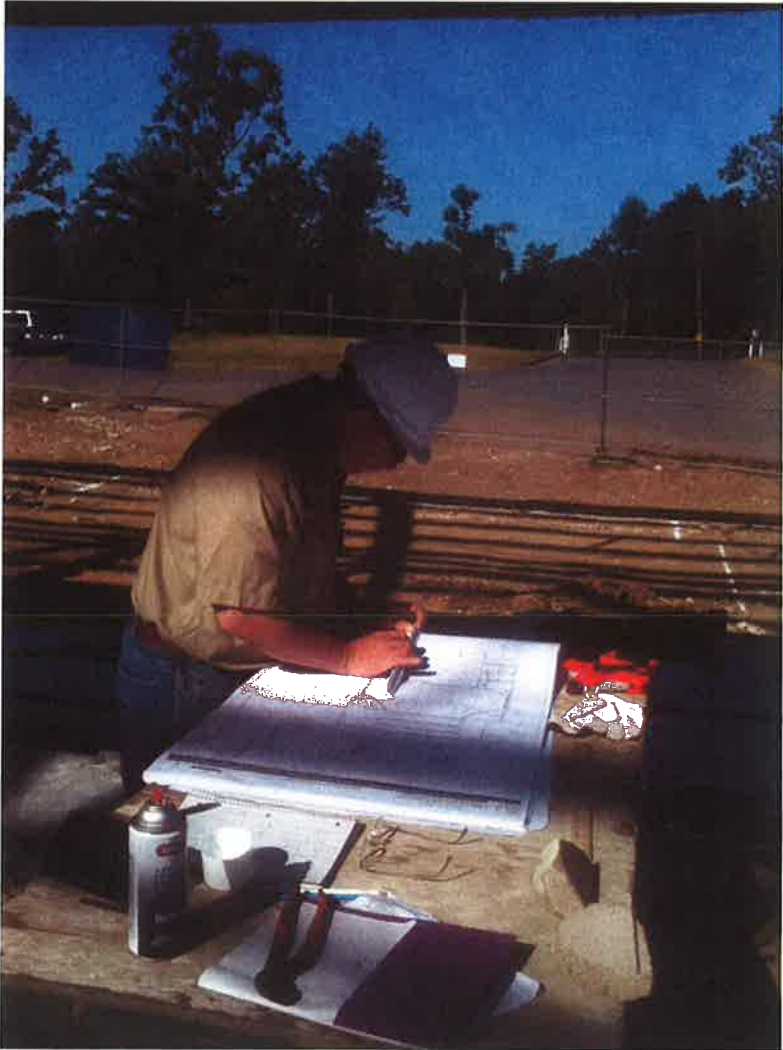
Mike Lawrence begins project layout, 2010 Auditorium Reconstruction, North Pulaski High School
