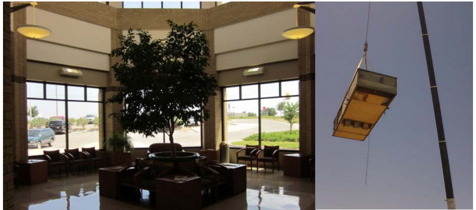
Phase 1 Rooftop Unit Replacement
