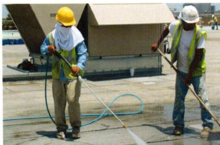
Roofers begin the process by power washing the existing surface.
