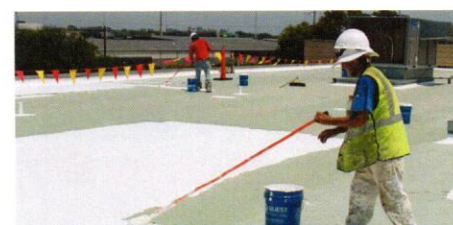
Almost done! Applying the final coat.
