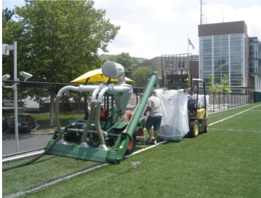
BADGER Machine Removing Turf Infill into Super Sacks on Site (Georgetown Day School, Washington, D.C. 2009). The BADGER uses high pressure air jets and a suction system to remove intill.
