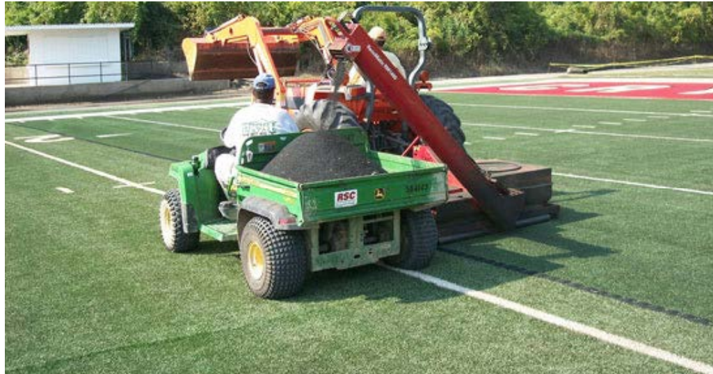
RENOMATIC Machine Removing Turf Infill—Note rubber pile in tractor bed
