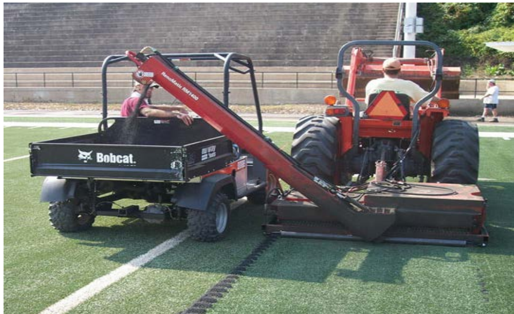
RENOMATIC Machine Removing Turf Infill, El Paso, Texas, 2009. The RENOMATIC machine uses a combination of aggressive agitation and suction to remove infill particles.
