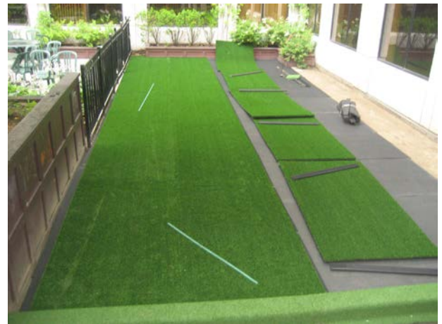
AstroMod installation, mid installation
