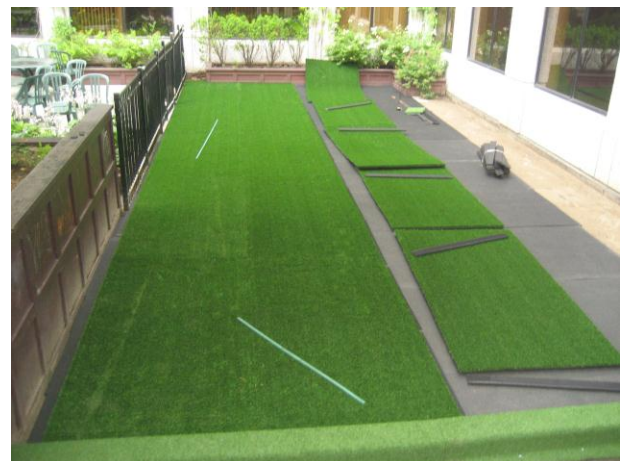
AstroMod installation, mid installation
