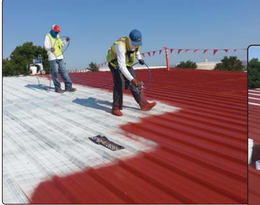
Spraying on Apoc 291 Rust Inhibitive Primer
