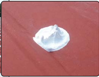
Sealing fasteners with Apoc 264
