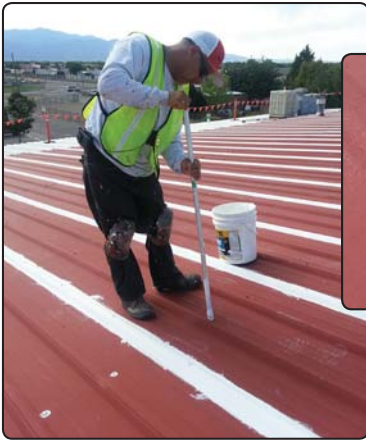
Sealing fasteners with Apoc 264
