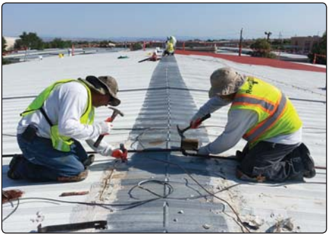
Removing old material used on previous repairs
