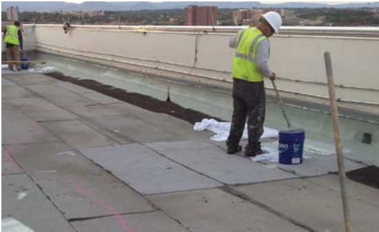
Applying the PremiumCoat® System to the existing mod bit roof
