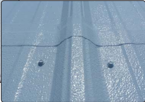
Close up of 1st coat of Apoc 252 SunGrey
