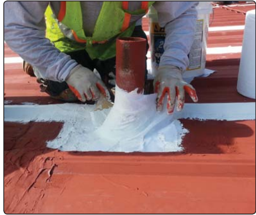
All perimeters, curbs and penetrations are sealed with Apoc 264 & reinforcing fabric
