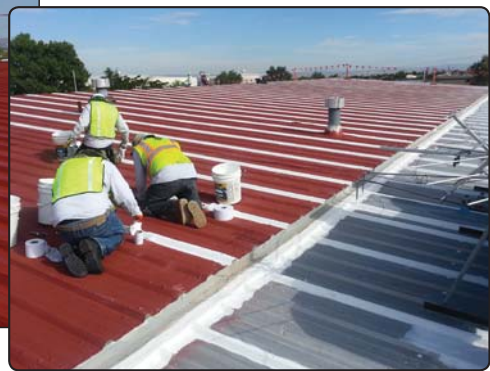
Sealing vertical seams with Apoc 264 Flash and Seal and polyester reinforcing fabric
