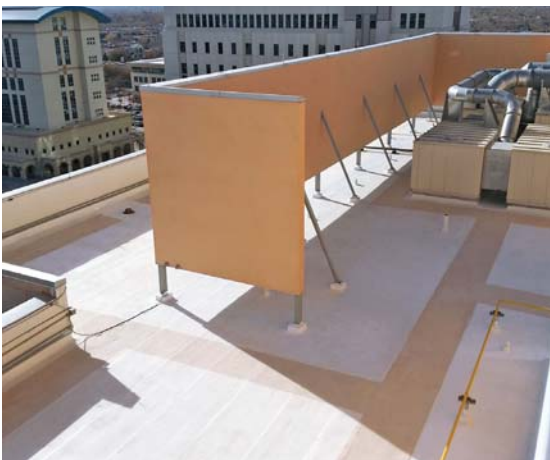
TrafficCoat, a non-skid surface, was used to clearly mark rooftop walkways
