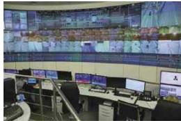
▲ A control center can monitor the remote tunnel traffic by long distance and real-time video data transmission.
