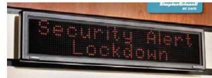
The Simplex TrueAlert Display is a UL-Listed IDNet addressable device that is controlled, monitored, and powered by one or more Simplex 4100U fire alarm panels. The True Alert text messaging appliance displays automated emergency messaging but allows custom end user messages to be displayed as well. Informative end user messages are overridden in the case of an emergency and a designated emergency message is displayed.
