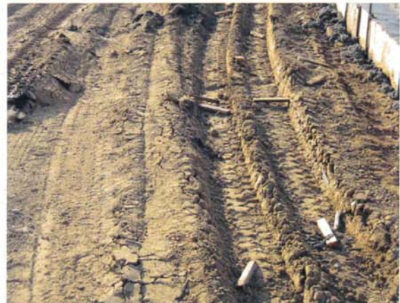
Example of failed subgrade
