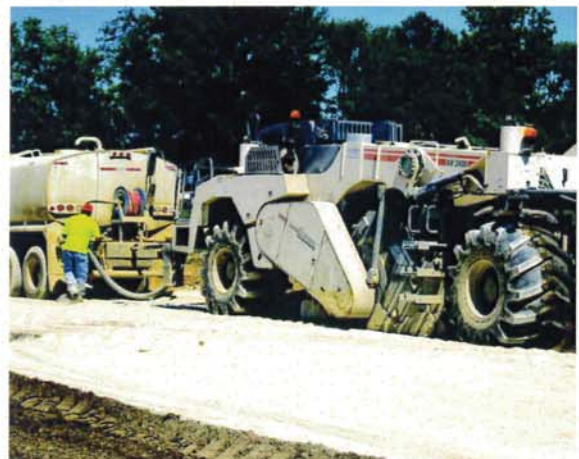
Soil stabilization in process
