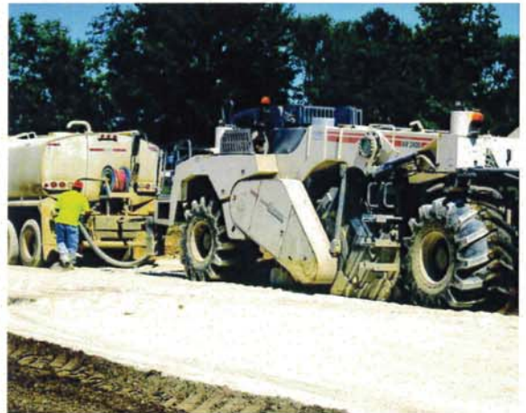
Soil stabilization in process
