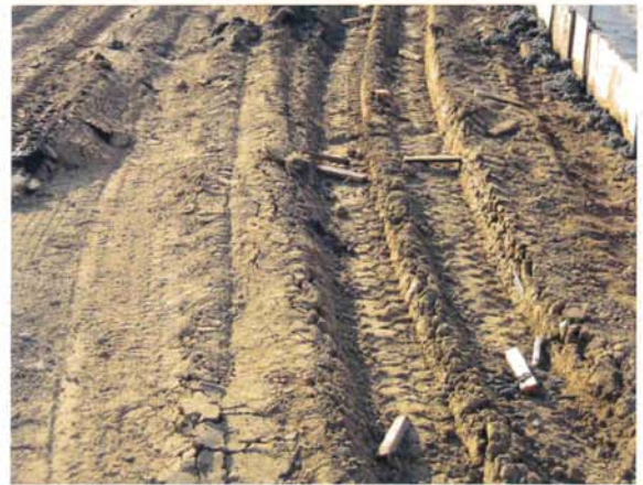
Example of failed subgrade
