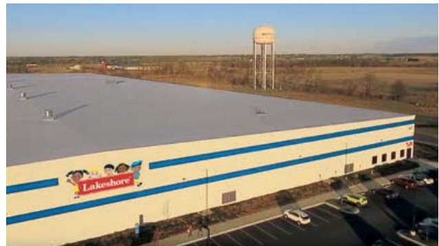
Our eastern distribution center in Midway, Kentucky.
