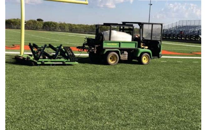
3- decompaction with re-leveling
