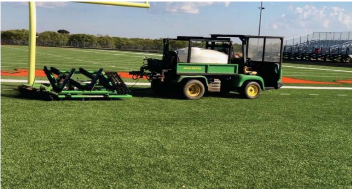
8 - Re-level & final groom
