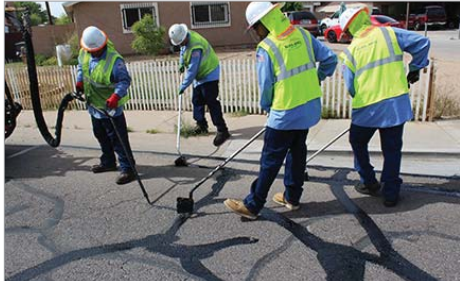
CRACK SEALING
