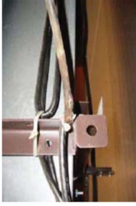
Electrical Wiring Issues
