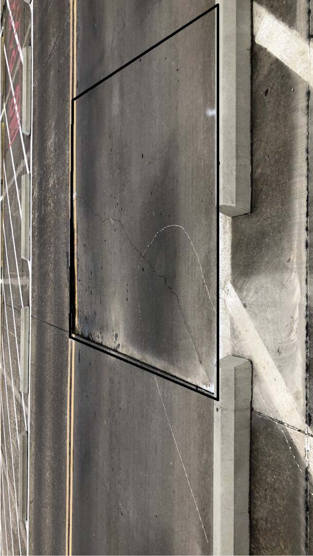
Area 5 – 12.5' X 7.5' - We recommend replacing half of this panel as it is likely failing further than the markings indicate.
