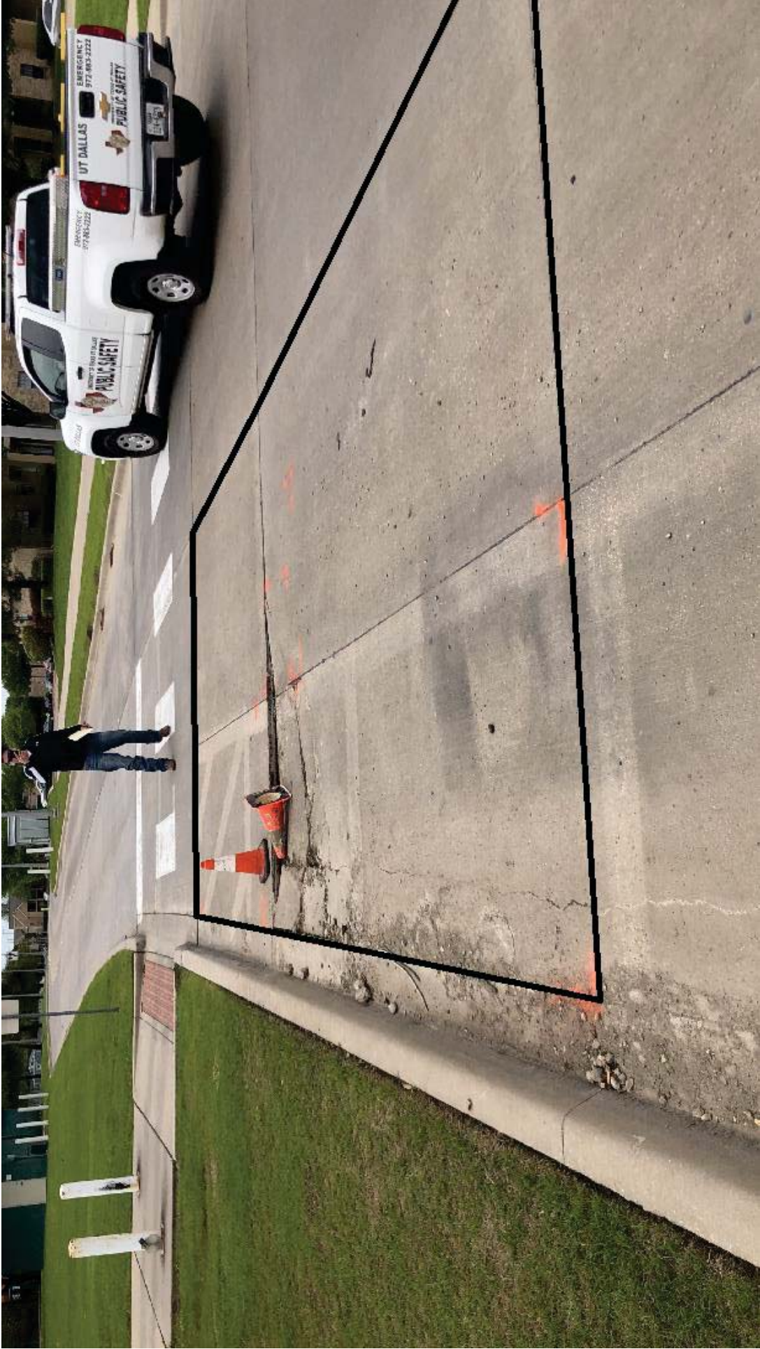
Area 10 - 12' X 26' Recommended to replace full panels at this location
