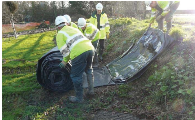
An existing launch point
