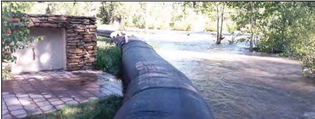
More 3' and 4' high AquaDams® used for flood protection in Sun Valley, ID.
