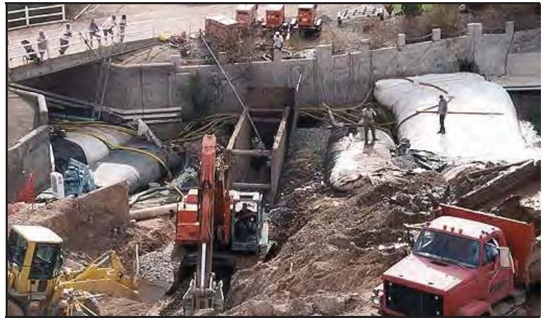
8' and 4' high AquaDams® used to dewater for "open cut" pipeline repair in Parker, AZ.
