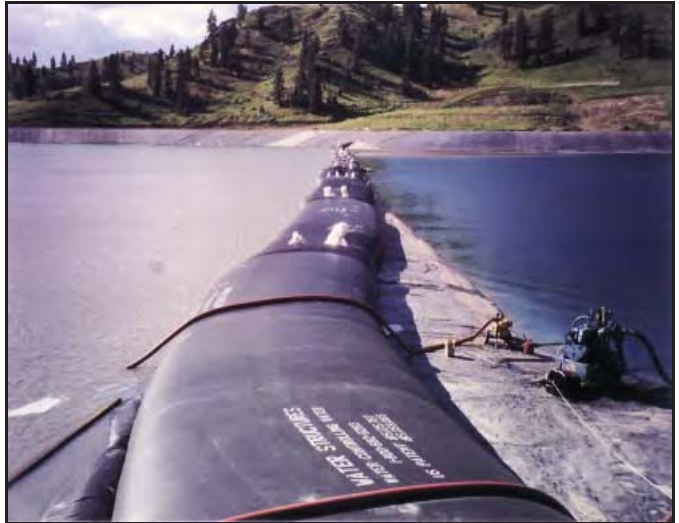
1,300 linear feet of AquaDams® in an arsenic pond, Northern WA.
