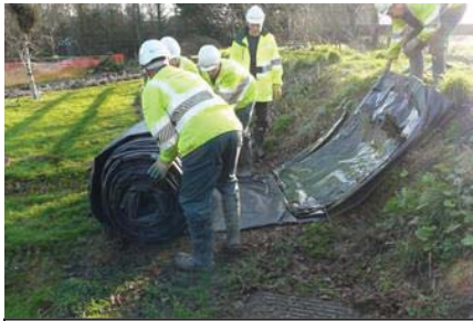
Existing launch point e.g. flood bank
