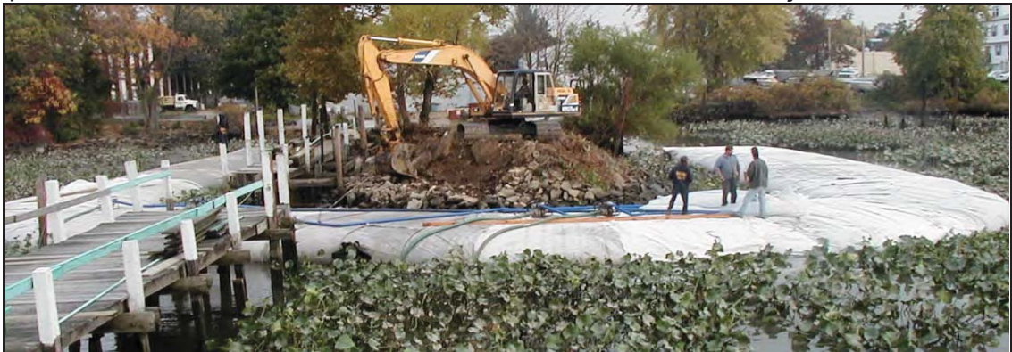
8' high AquaDam® used to isolate a work area for pier construction in Philadelphia, PA.
