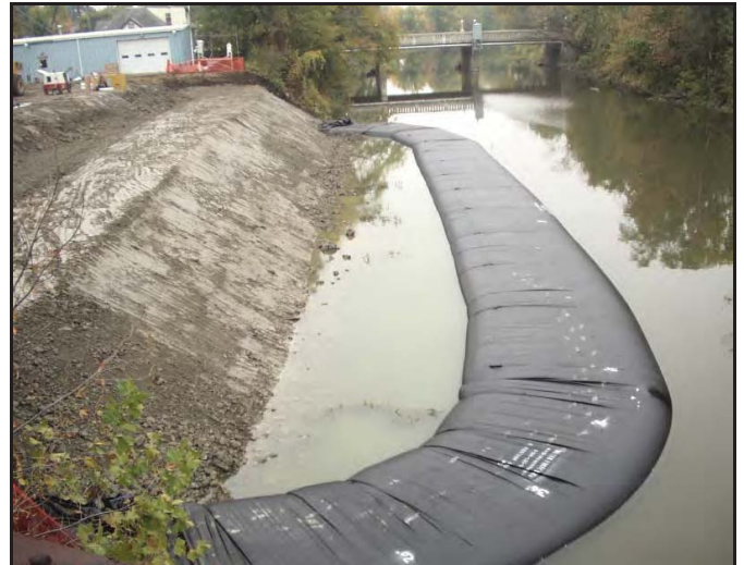
AquaDam® being used to isolate the Vermilion River from contaminants, Pontiac, IL.
