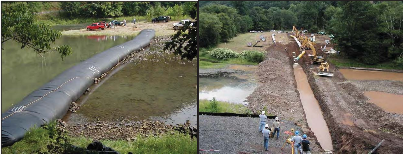
4' high AquaDams® were used upstream and downstream of this trench to contain sediments during a Williams Transco gas pipeline installation in Pine Creek, Williamsport, PA.
