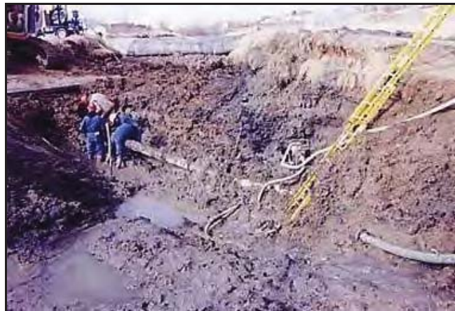
AquaDam® blocks canal in Denver, CO
