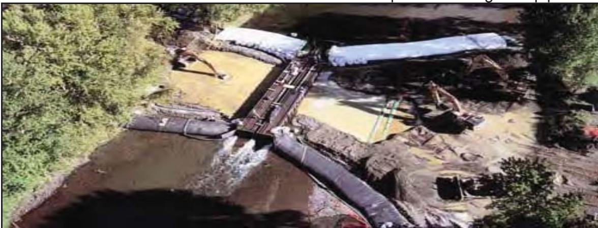
8' and 6' high AquaDams® abut into the sides of a flume near Grand Forks, BC.
