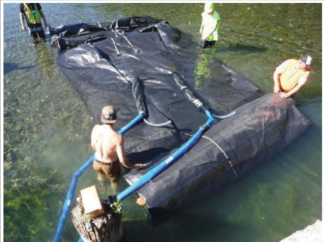
Two blue-color hoses are used to fill the two AquaDam inner tubes
