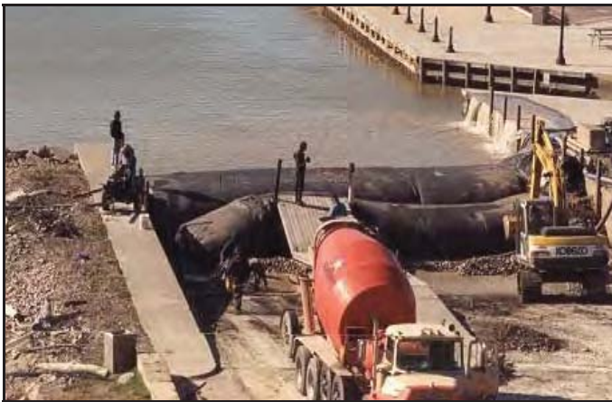
AquaDams®, used to dewater for boat ramp repair on Lake Erie, OH.
