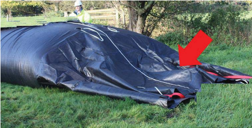
Joining collar attached to the end of each 25m AquaDam
