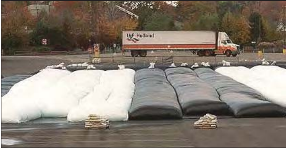
4' and 5' high AquaDams® used for salt water storage during cleaning and renovation of Shamu the killer whale's tank at Sea World Ohio.
