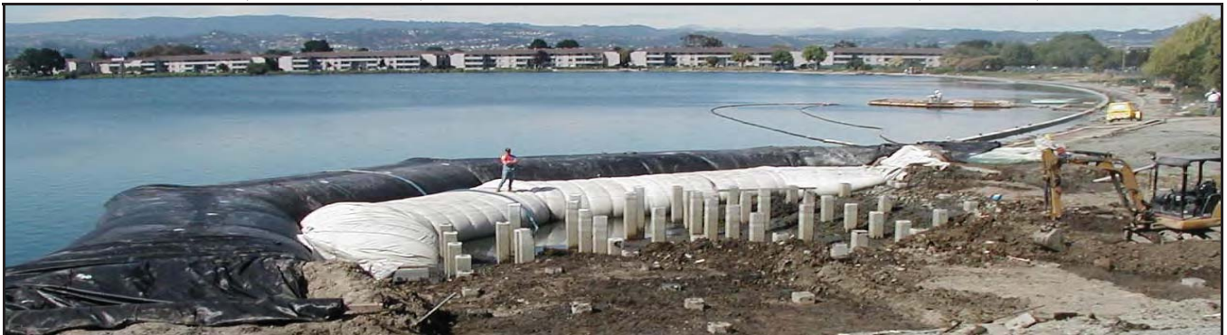
Dewatering for amphitheatre construction, Foster City, CA.
