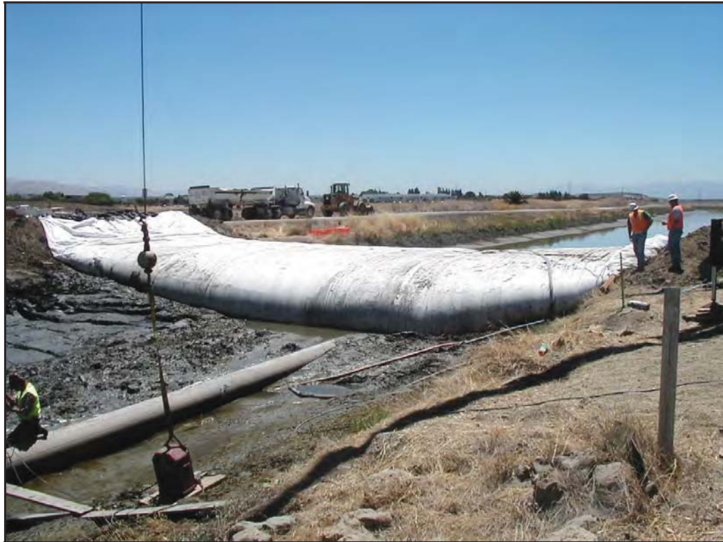
14' high AquaDam® used to dewater a tidal canal in Fremont, CA.
