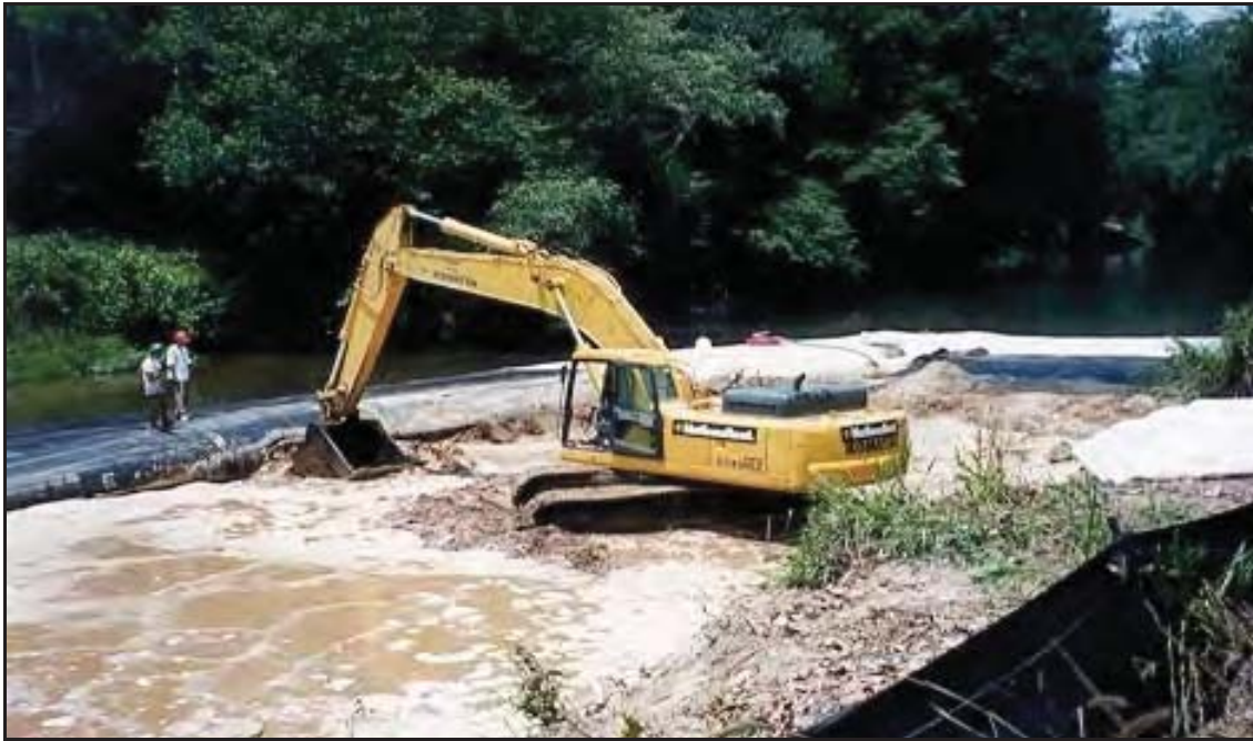
8', 6' and 4' high AquaDams® used to contain sediments during a Williams Transco natural gas pipeline repair project on the Bogue Chitto River, McComb, Mississippi.
