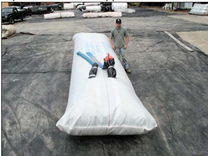
2. Fill tubes extend out the top. The AquaDam is inflated with air.
