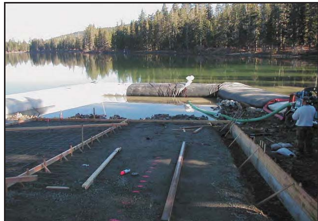
AquaDams® used to dewater for boat ramp construction on Gold Lake, CA.
