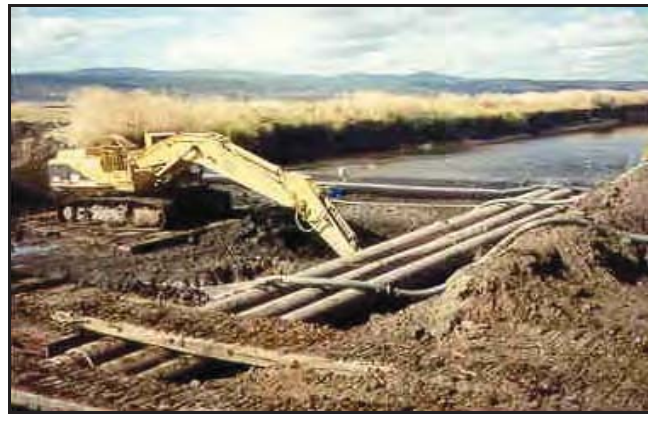
6' high AquaDams in the Pitt River, CA. The river passed through the pipes.
