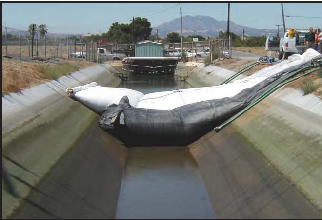
8' and 5' high AquaDams®, used to dewater a canal for pump station repair, Antioch, CA.
