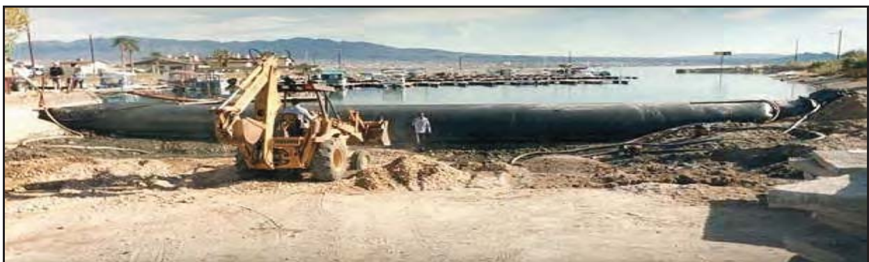
6' high AquaDam® in Lake Havasu, CA, along the Colorado River.
