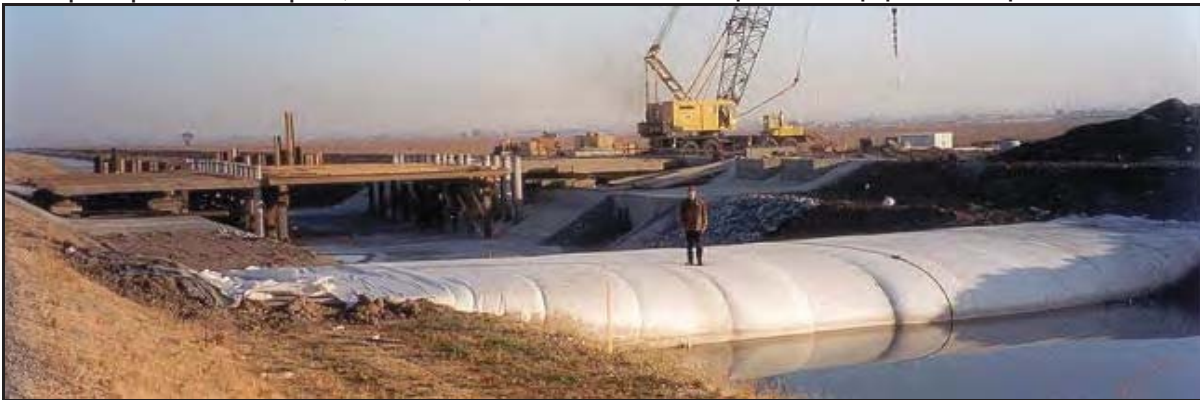
10' high AquaDam® used to dewater for bridge pier construction, Sacramento, California.
