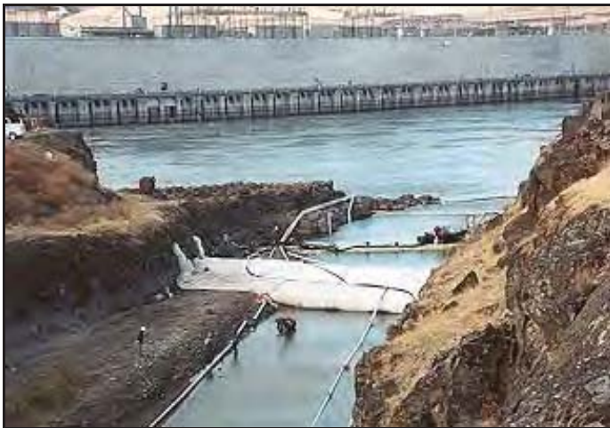
Containing a chemical spill on the Columbia River, The Dalles, OR
