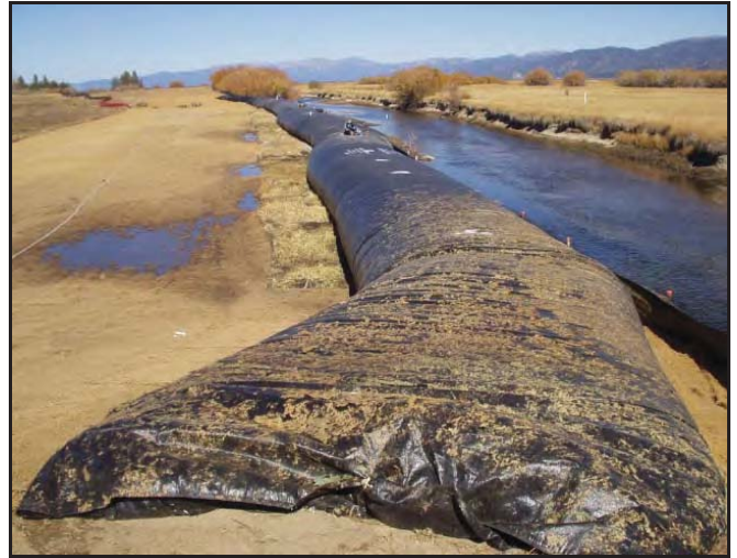
4' high AquaDams® used to separate the Upper Truckee River from newly created wetlands to prevent erosion into Lake Tahoe, Lake Tahoe Keys, CA.
