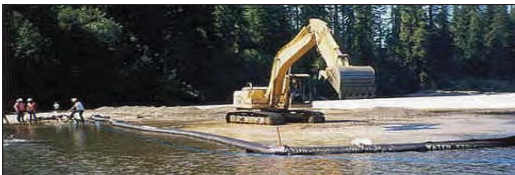
Fish habitat construction on the Eel River, Redcrest, CA.
