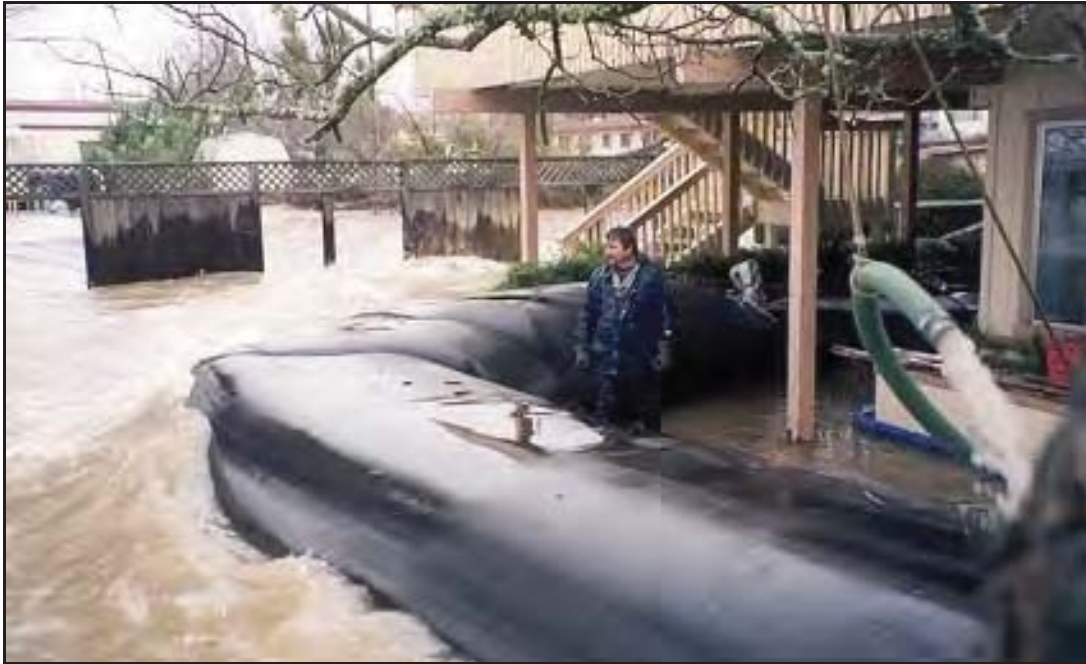
3' high AquaDams® being used for homeowner flood protection in Clear Lake, CA.
