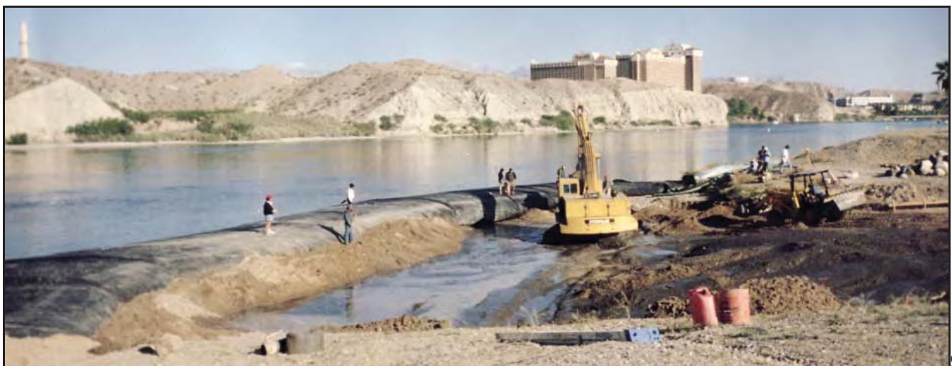
high AquaDam® used for boat ramp construction in Bullhead City, CA.
