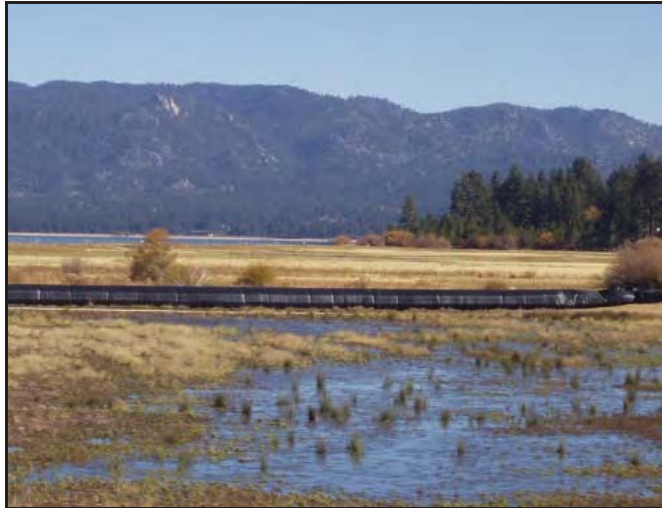
4' high AquaDams® used to separate the Upper Truckee River from newly created wetlands to prevent erosion into Lake Tahoe, Lake Tahoe Keys, CA.
