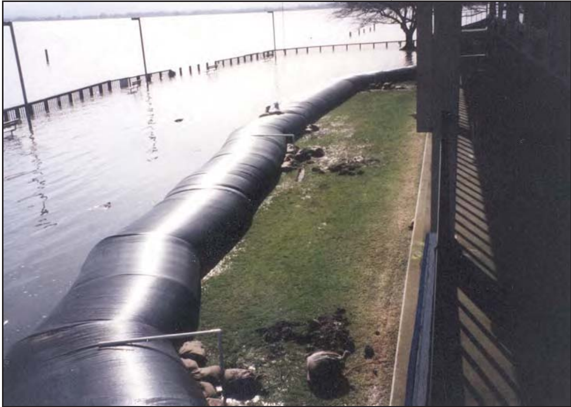
4' high AquaDams® used for flood protection of the Skylark Hotel in Clear Lake, CA.
