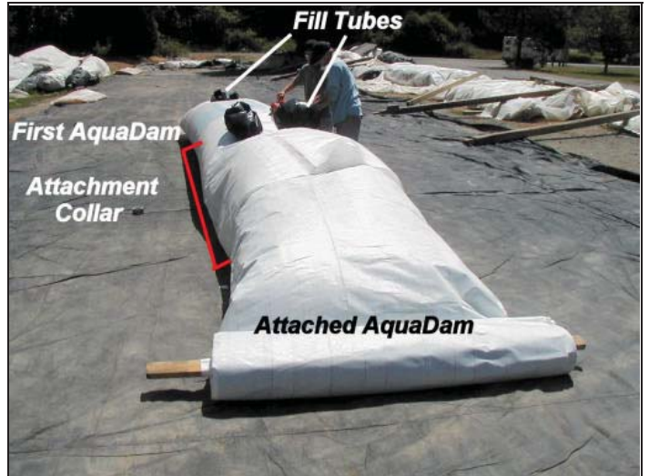
4. Two AquaDams being connected together using the attachment collar.
