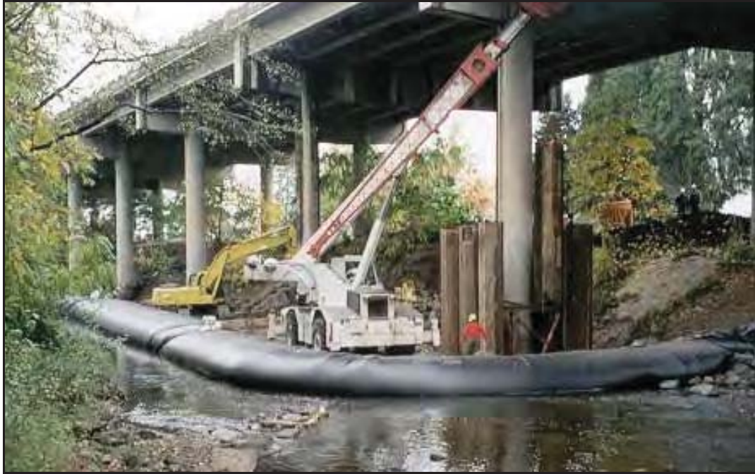
Several 6' high AquaDams® used to dewater a bridge pier for retrofitting in Bear Creek, Medford, OR.
