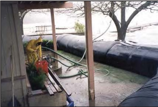
3' high AquaDams® being used for homeowner flood protection in Clear Lake, CA.
