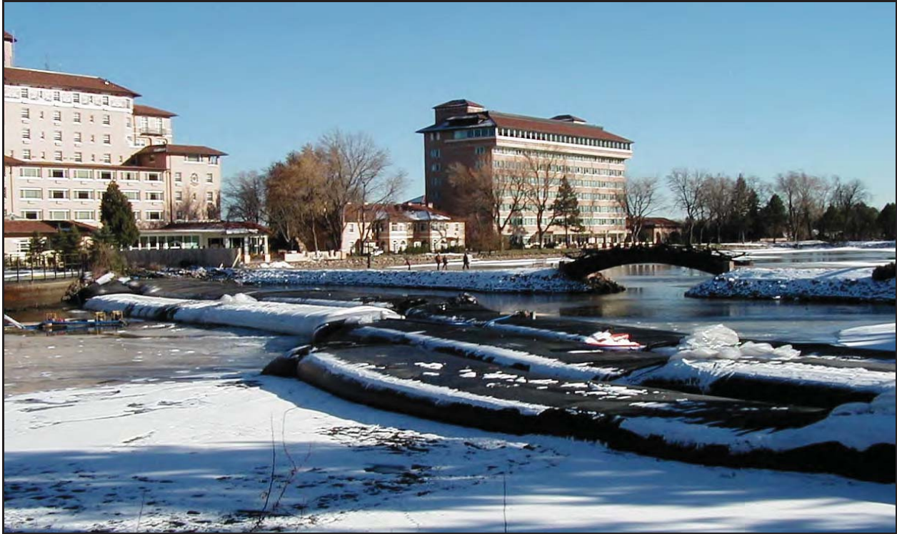
A combination of 8' and 14' high AquaDams® used to isolate and dewater one section of a lake separating two building complexes at the Broadmoor Hotel, Colorado Springs, CO
