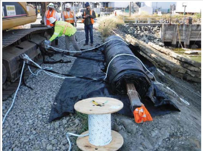
8ft tall, 100ft long AquaDam sits at the top of the starting bank
