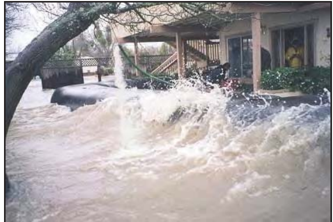
3' high AquaDams® being used for homeowner flood protection in Clear Lake, CA.
