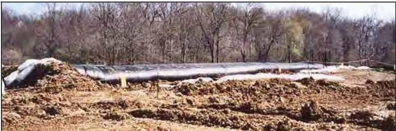
6' high AquaDam® used to store low-level radioactive water for Westinghouse in Northern PA.
