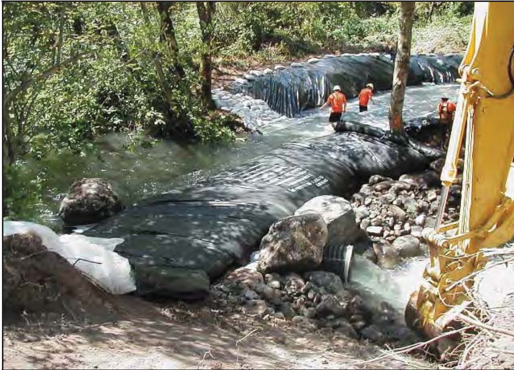
5' high AquaDam® used to divert water for installation of an irrigation check dam in Apple Creek, OR.
