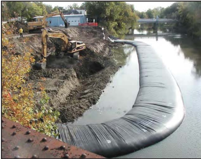
AquaDam® being used to isolate the Vermilion River from contaminants, Pontiac, IL.
