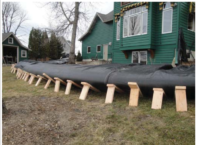
Many 2-board braces are in place along the side of the partially filled AquaDam.
