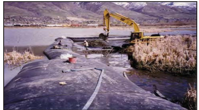
Wetland construction, Great Salt Lake, UT
