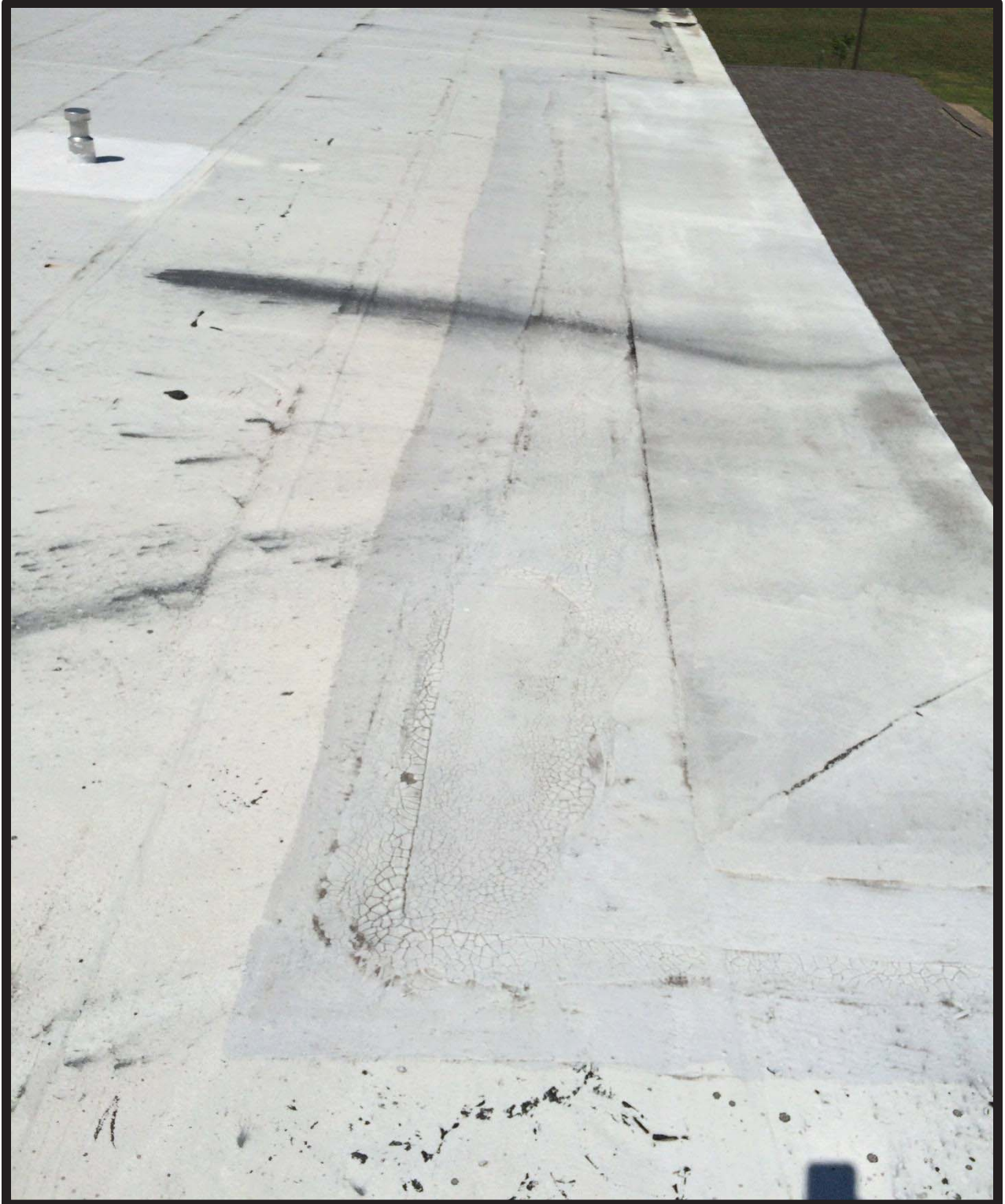
The Conference for the Seventh-Day Adventists, Alvarado, TX. Existing roof is a 10 mil acrylic coating over modified bitumen cap sheet. Multiple leaks throughout the building.
