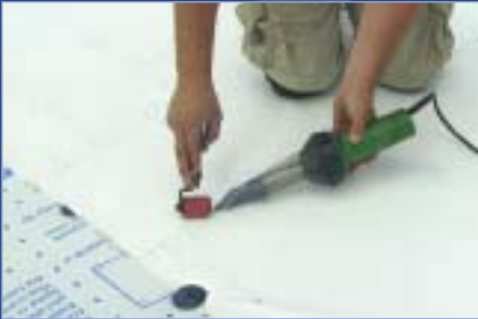
Roof installation in Saginaw, Michigan.
