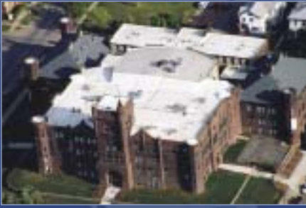
Castle On The Hill in Sioux City, Iowa Installed by Nohava Construction, Co.
