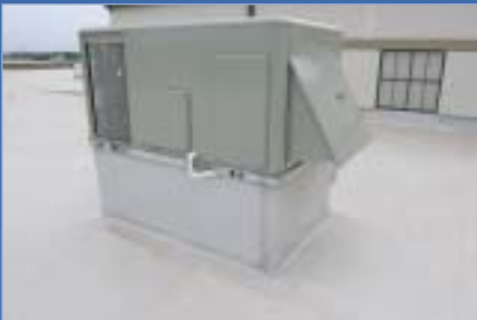
HVAC unit installed in Alma, Michigan.
