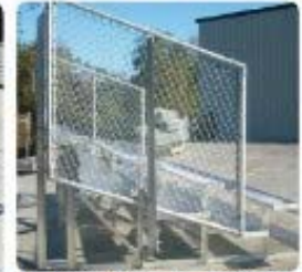
Chain Link Guardrail
