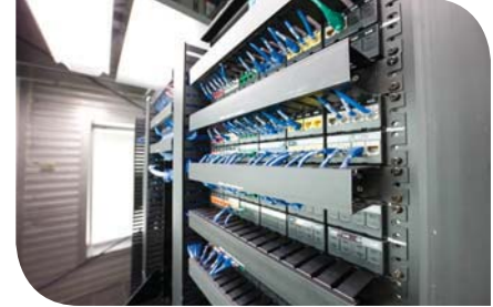
Quality Infrastructure Installation
