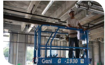
24/7 Lighting & Electrical Service
