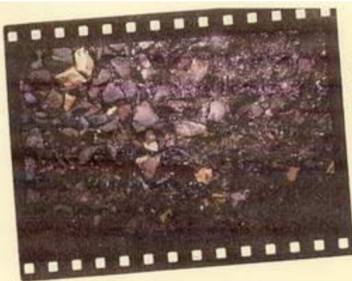
Figure 3 At 40x magnification, this photo of a glass-reinforced laminate shingle displays foot traffic damage. With close examination of the granules and surface asphalt, one can see that the granules have been extracted from their original embedment in the surface coating, consistent with typical foot traffic.
