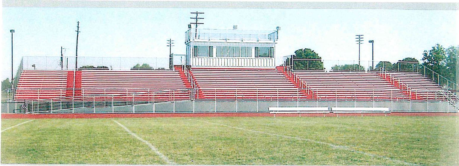
New Lebanon High School - Lebanon, OH
