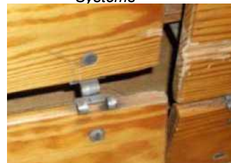
Broken Skirt Board Hinges
