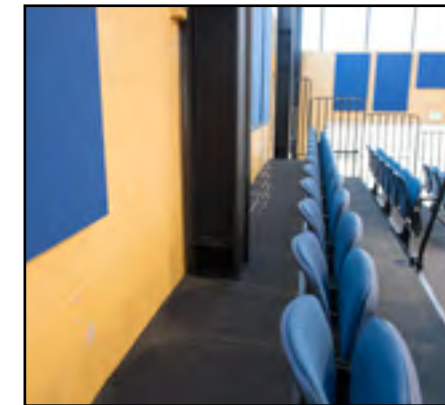
Building Column Cutouts
