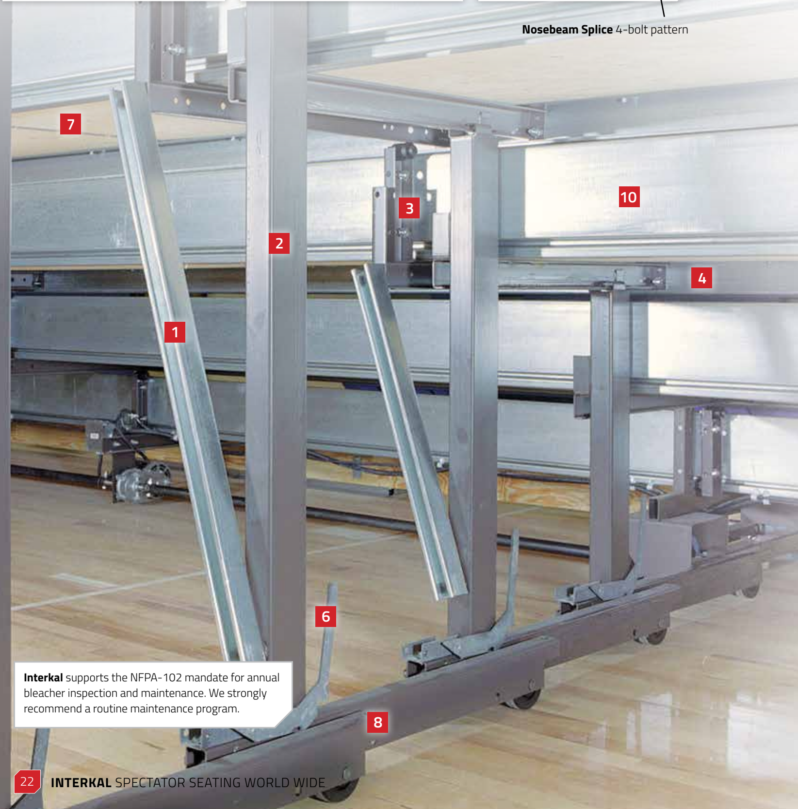
Riser Splice 8-bolt pattern
