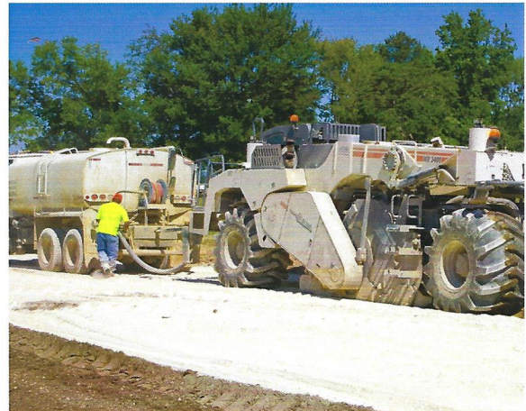
Soil stabilization in process
