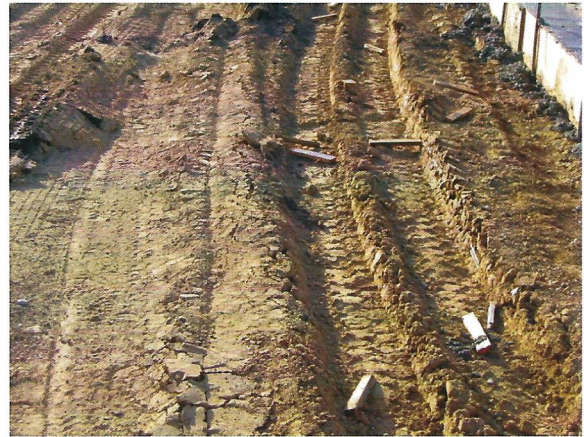
Example of failed sub grade
