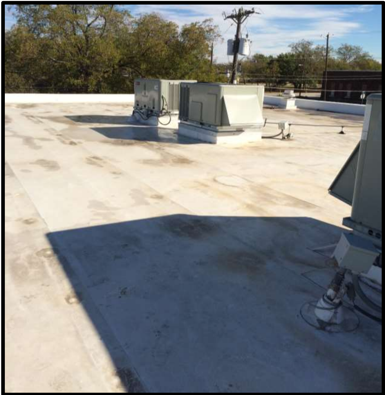
Anna, Texas Police Department before silicone. Existing roof was a deteriorated TPO roof with multiple roof leaks.
