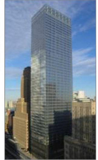
7 World Trade Center Integrated security system
