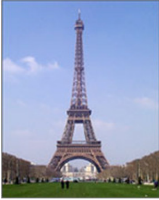
Eiffel Tower Fire detection & extinguisher systems
