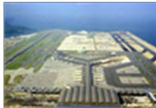
Hong Kong Int'l Airport Security system
