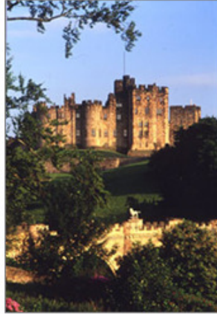
Alnwick Castle Extinguishers
