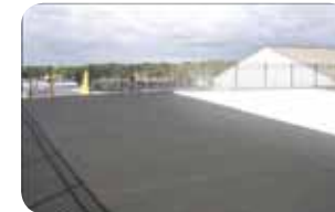
Roof Restoration Systems
