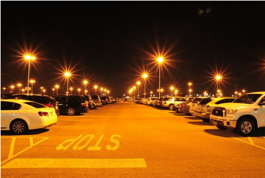
Old YELLOW 1130 watt low sodium vapor lights
