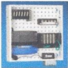
Media Distribution System
