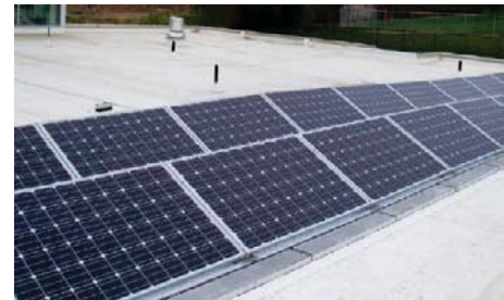
Solar for Schools is expected to remove more than 8,000 tons of carbon dioxide from the atmosphere over 20 years, equivalent to the carbon offset that would be generated by planting 11,000 trees and letting them grow for ten years.
