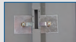
User doors reinforced at latches
