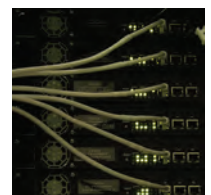
Network connections into SVSi's Windowing Processors
