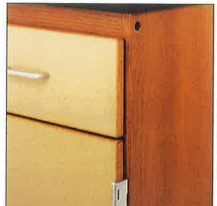
PLASTIC LAMINATE; 3MM OAK EDGE BAND, PARTICLE BOARD CORE, PARTIAL OVERLAY
