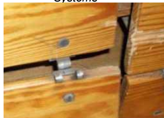
Broken Skirt Board Hinges
