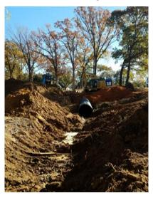
The project included removal of an existing concrete golf cart bridge, 150 LF of golf cart path, three large trees and stumps; the installation of 80 LF of new 36" culvert pipe, and associated headwalls, exit rock riprap, 180 LF of new cart path; and compaction of 150 CY of select fill.
