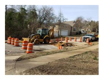
Repairs of similar nature were completed at an adjacent inlet box. Including removing several feet of fill using a hydrovac, forming a new concrete collar, compacting, and regrading the affected area.
