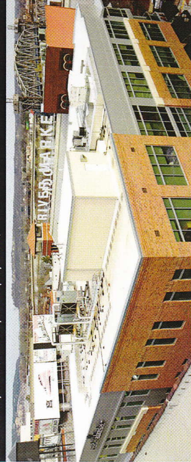
Little Rock River Market Arcade Building TPO Roof System (Thermoplastic polyolefin)
