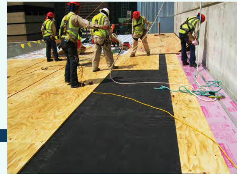
In these photos different layers of the metal deck, the insulation, the cement board, structural plywood and the acoustic mat can be seen
