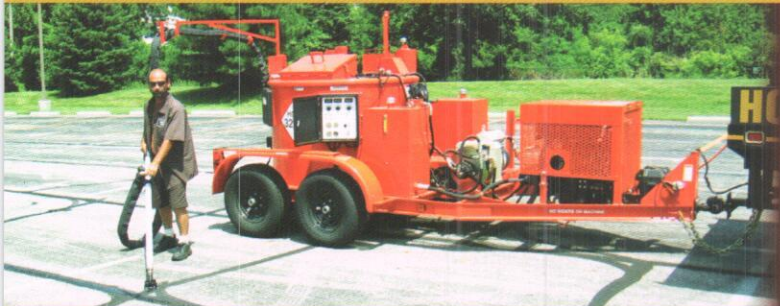
Cracksealing
