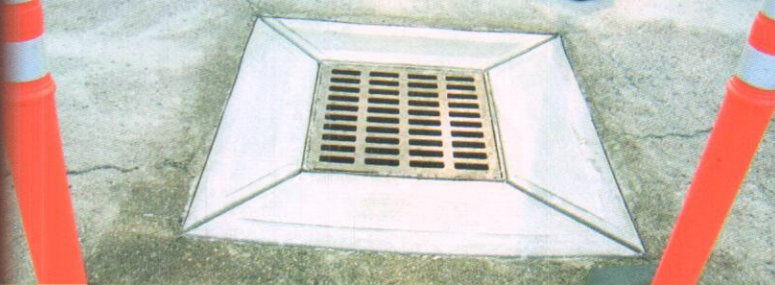
Concrete and Catch Basins
