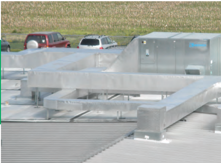
Mechanical upgrades including Energy Recovery Unit to condition outside air
