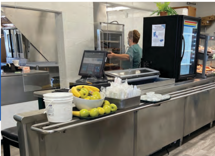
Kitchen renovations including flooring, painting, and all new kitchen equipment
