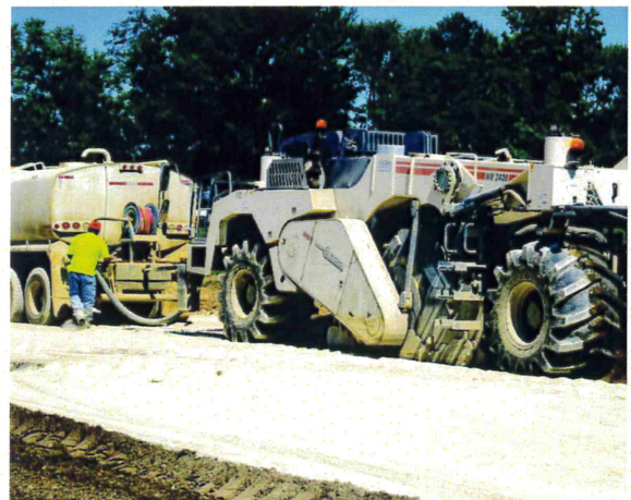
Soil stabilization in process
