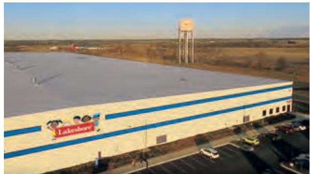
Our eastern distribution center in Midway, Kentucky.
