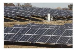
Johnson Controls also designed and constructed a 1,000 kW ground-mount PV system located at the Back River Waste Water Treatment Plant. Using SolarWorld modules and leveraging a grant from the Maryland Energy Administration, this project supports the City's objectives toward self-generation of 30% of all energy. This is a fixed-tilt, custom racking system suitable for the site's topography.
