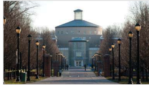
We installed a campus wide security system at CUNY – College of Stanton Island.
