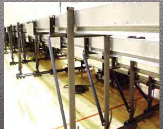
Above: 2400 Series bleacher understructure
