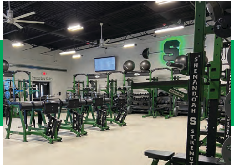
Design Build construction of new Weight Room
