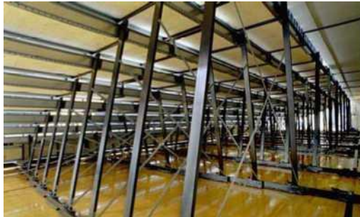
Safety Check List Below the Deck What to look for...
