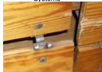
Broken Skirt Board Hinges
