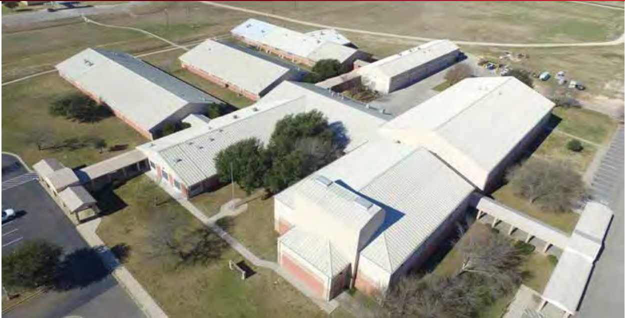
McGregor ISD - Installed in 2016
