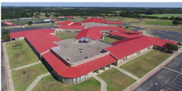
Bremond ISD - Installed in 2019
