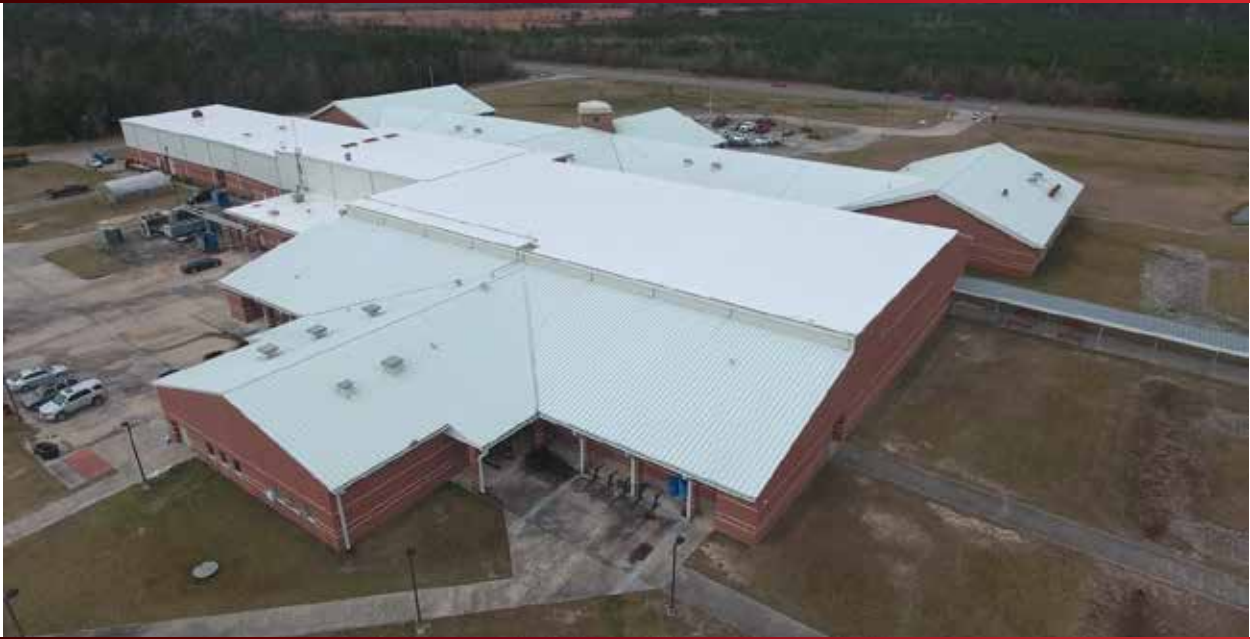
Groves ISD - Taft Elementary School - Installed in 2009
