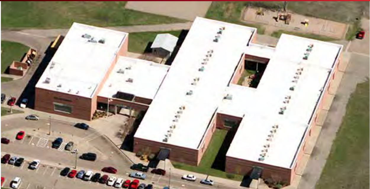
Waco ISD - Kendrick Elementary - Installed in 2010
