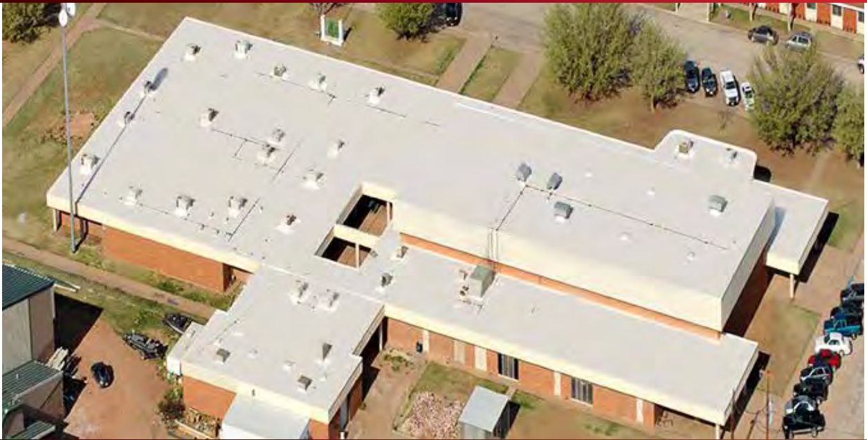
Cisco ISD - Elementary School - Installed in 2009
