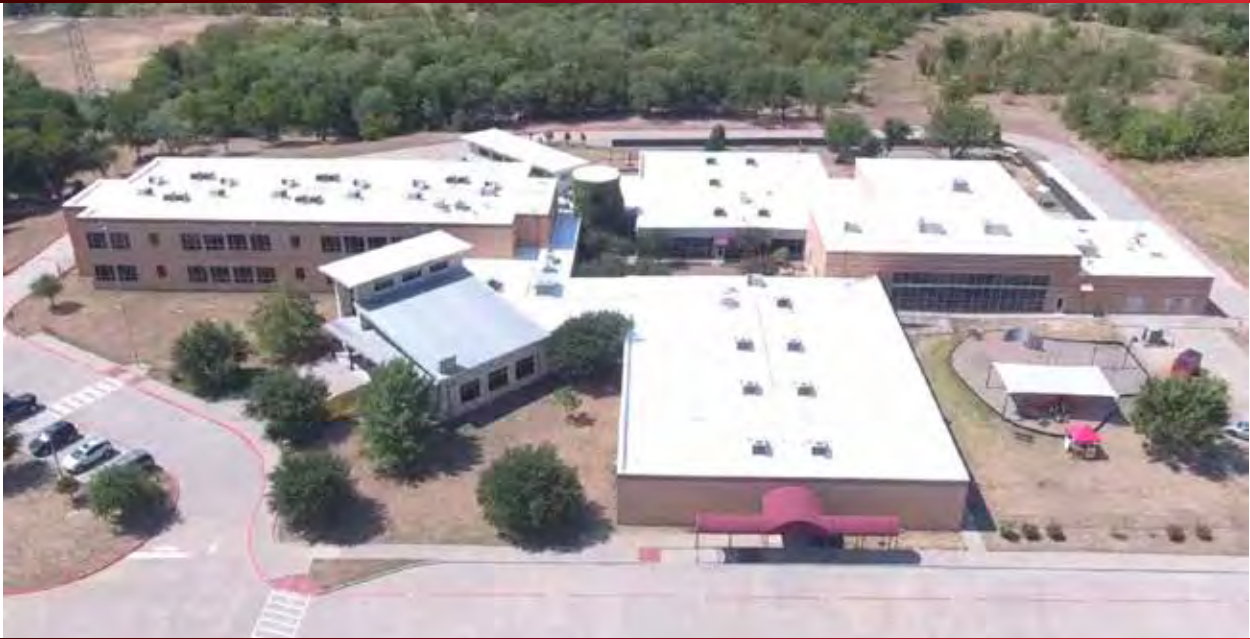
Maypearl ISD - Maypearl Intermediate - Installed in 2018
