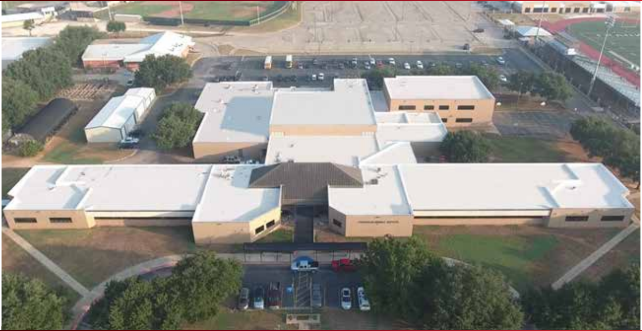
Oakwood ISD - Installed in 2007
