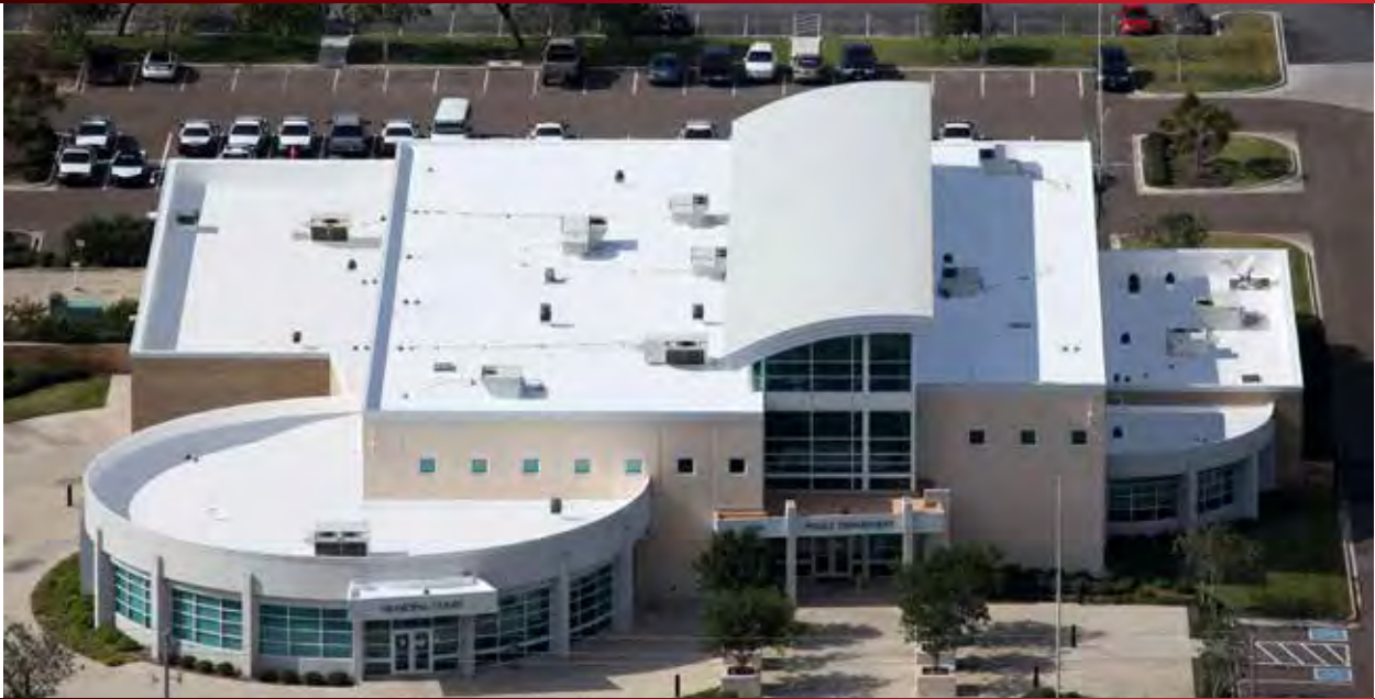
Pharr City Hall - Installed in 2009
