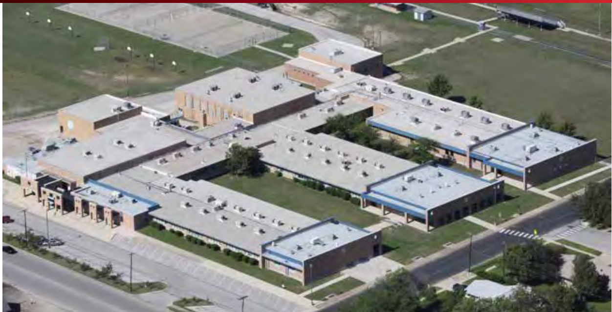
Killeen ISD Brookhaven Elementary - Installed in 2011
