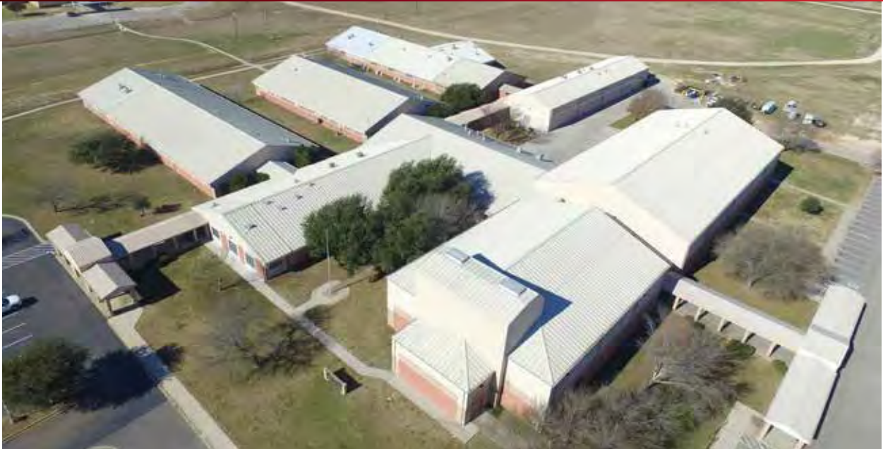
McGregor ISD - Installed in 2016
