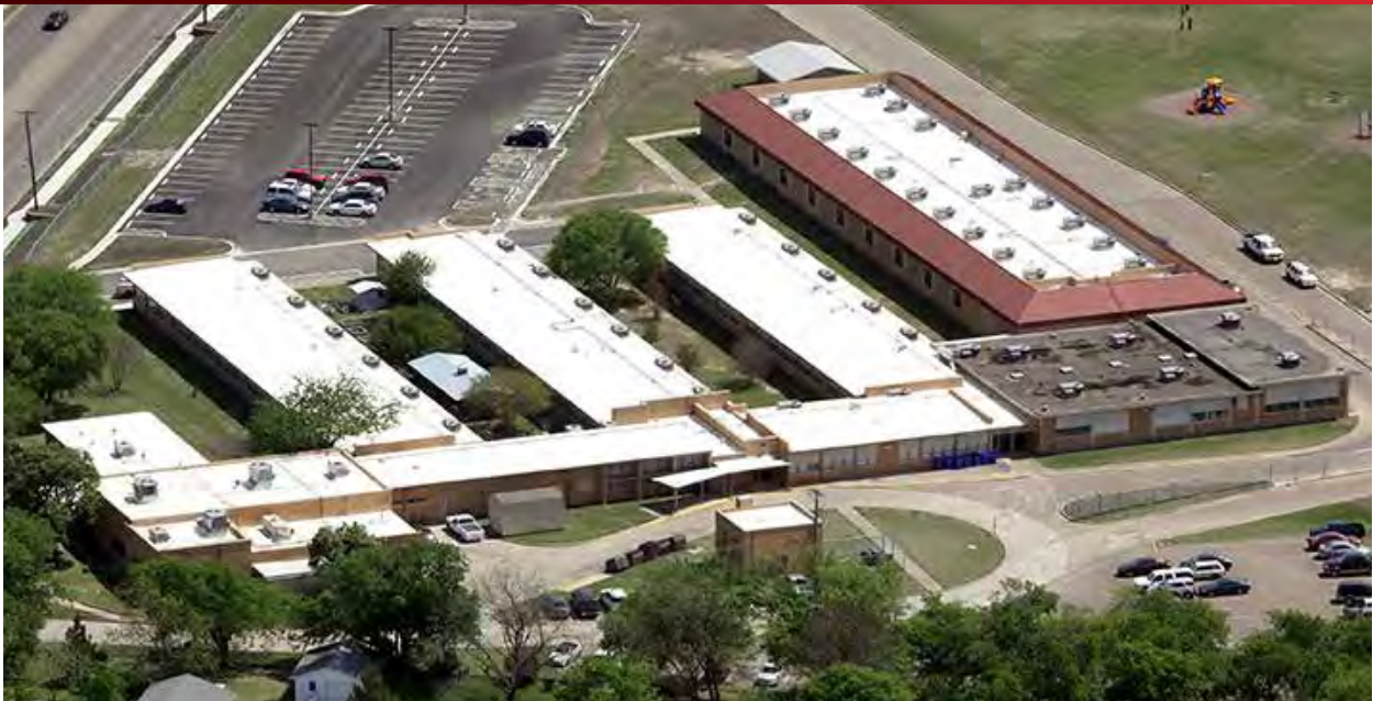
Waco ISD - Cedar Ridge Elementary - Installed in 2009
