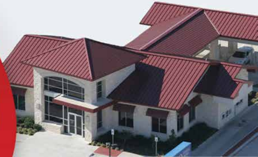
GENCO Federal Credit Union - Installed in 2005
