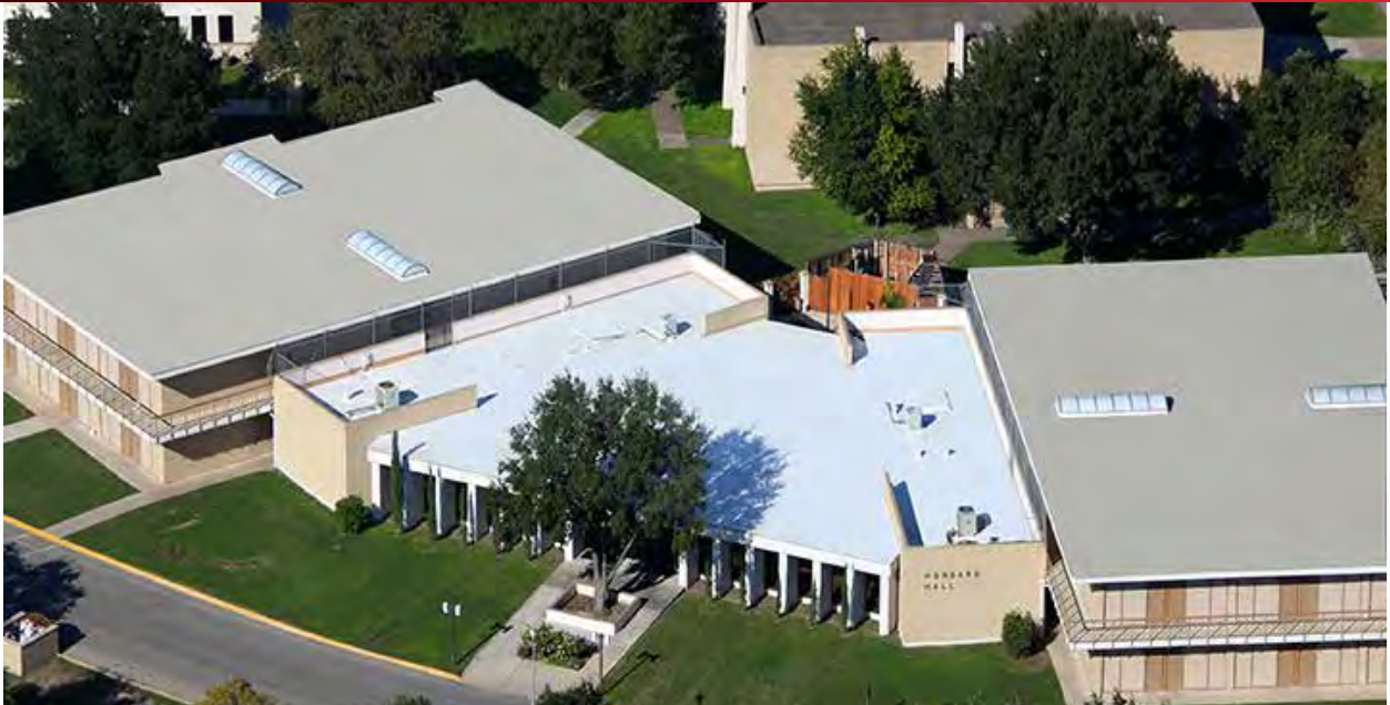
Odessa Sports Center - Installed in 2008
