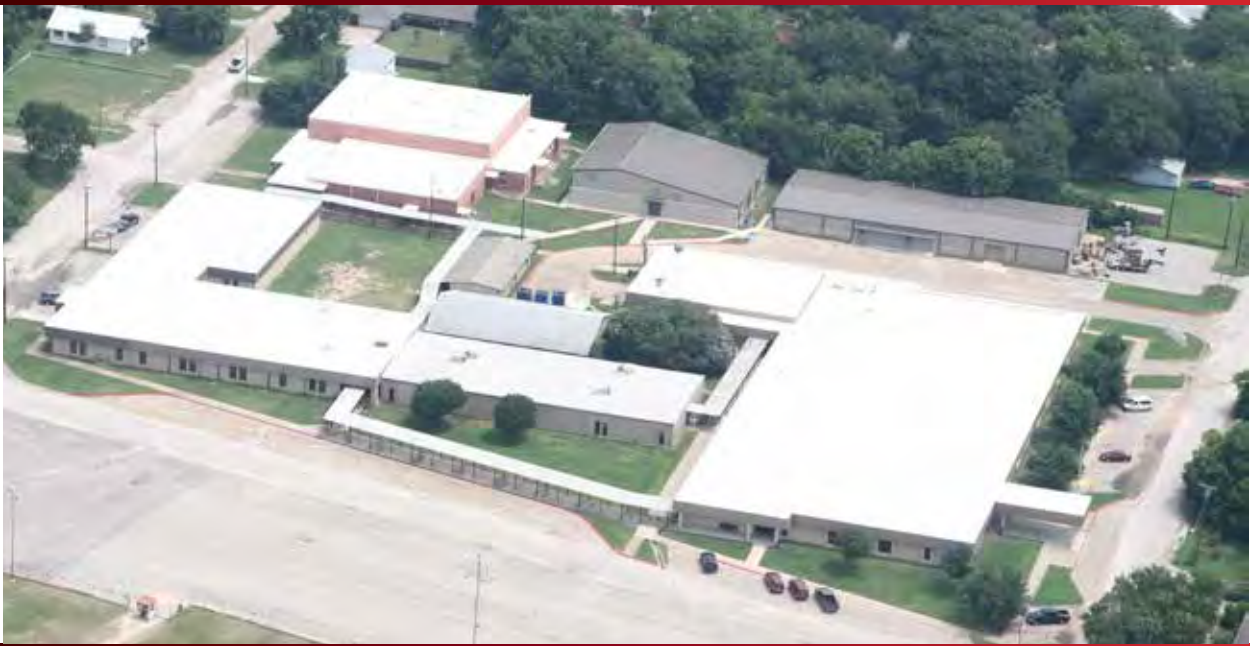
Connally ISD - Installed in 2007
