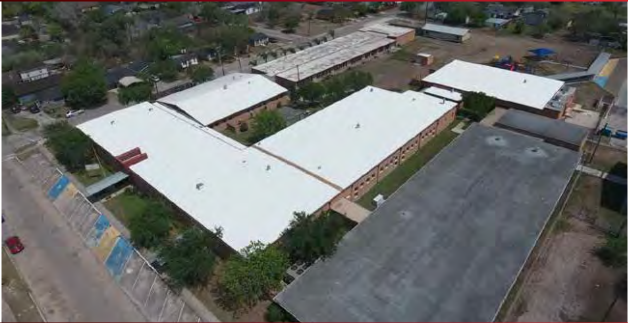
Santa Rosa ISD - Installed in 2014
