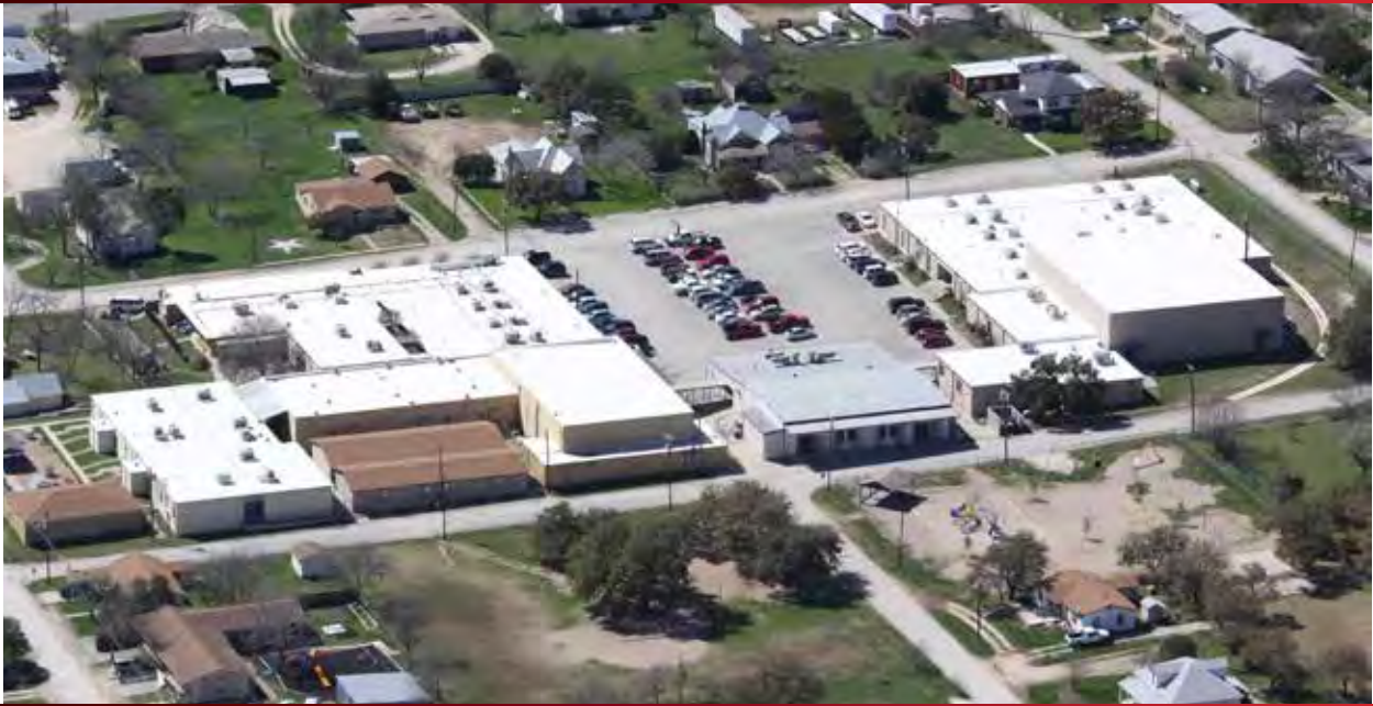
Jarrell ISD - Installed in 2018
