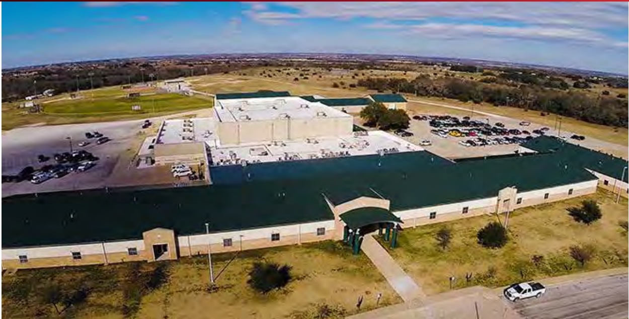
Dublin ISD - Installed in 2015
