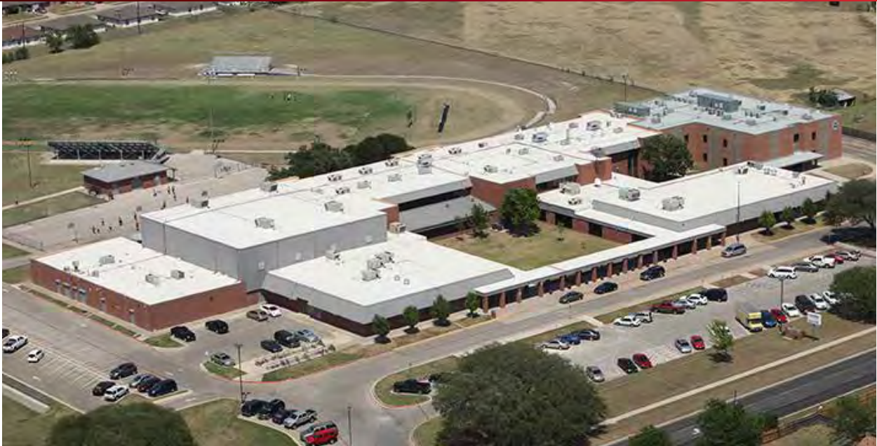
Killeen ISD Venable Village Elementary School - Installed in 2011
