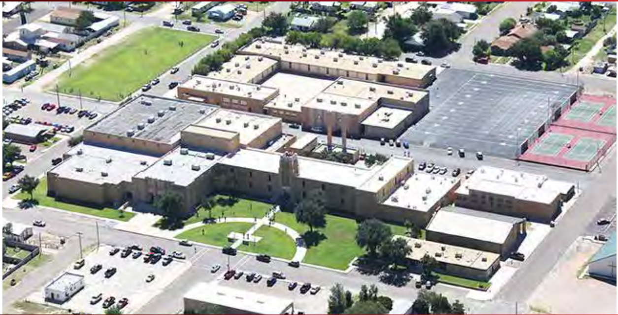
McCamey ISD - Installed in 2012
