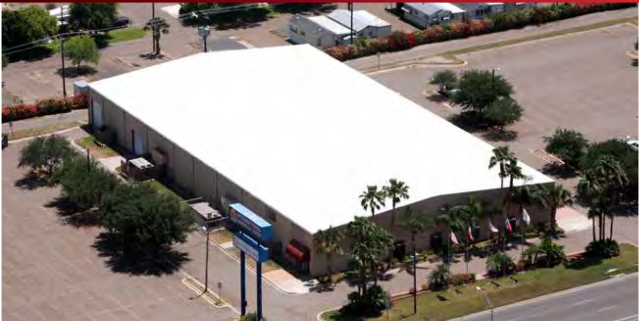
City of Arlington Facility Services - Installed in 2011
