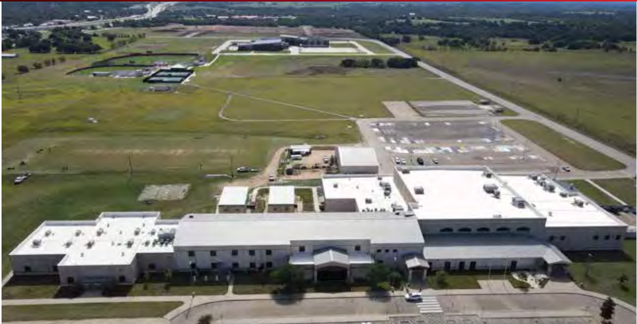
Troy ISD High School - Installed in 2020
